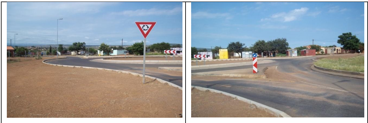
Scenes from the neighbourhood of Abundant grace. This is the Phase 4 traffic circle where the congregation is situated.
