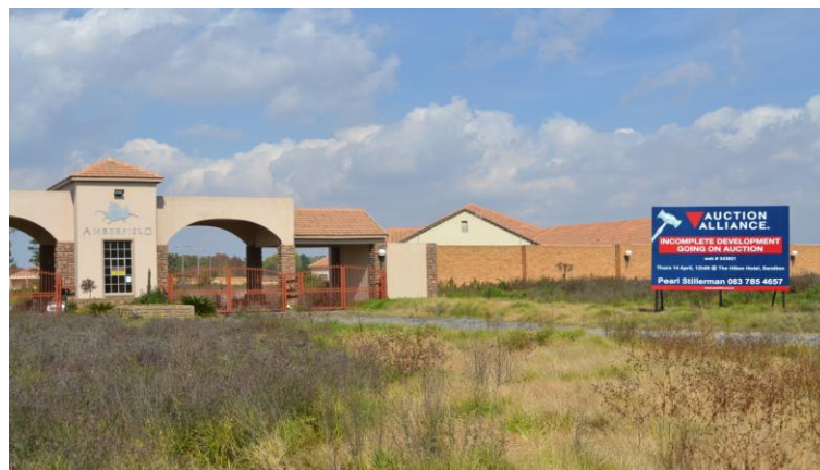
Photograph 4.1: The Amberfield retirement home. Source: Author (2011)
