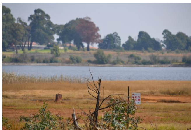
Photograph 2.3: Robinson dam in Randfontein. Source: Author (2011)
