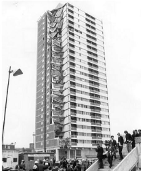
Figure 1.1: Ronan Point apartment building progressively collapsed after a gas explosion (Nair 2004)
