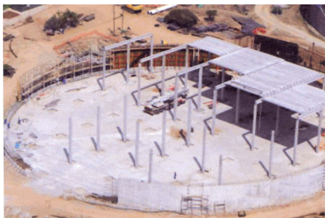
Figure 4.6: Parallel work in progress at the Polokwane reservoir (Concrete Trends 2010e)
