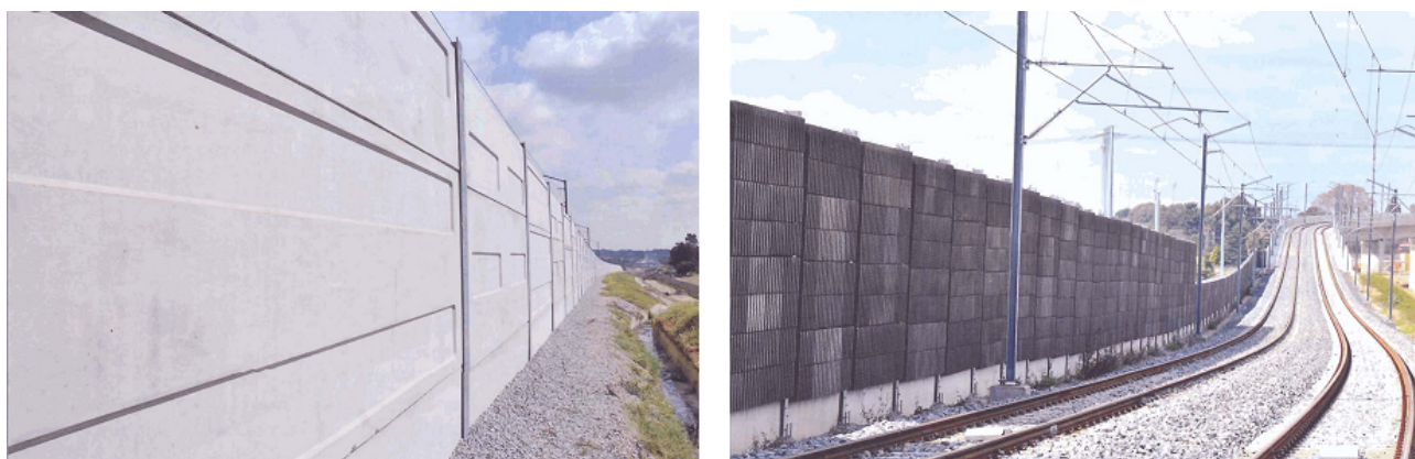
Figure 4.3: Normal precast walling (left) and absorption walling (right) is used as insulation barriers on the Gautrain project (Beer 2010)
