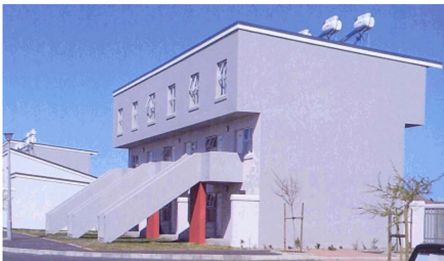
Figure 4.1: Steenberg social housing project (Lange 2011)
