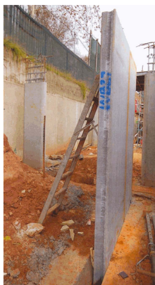
Figure 4.4: Hollow-core precast panels being propped into their footing positions at The Houghton hotel (Civil Engineering 2008a)
