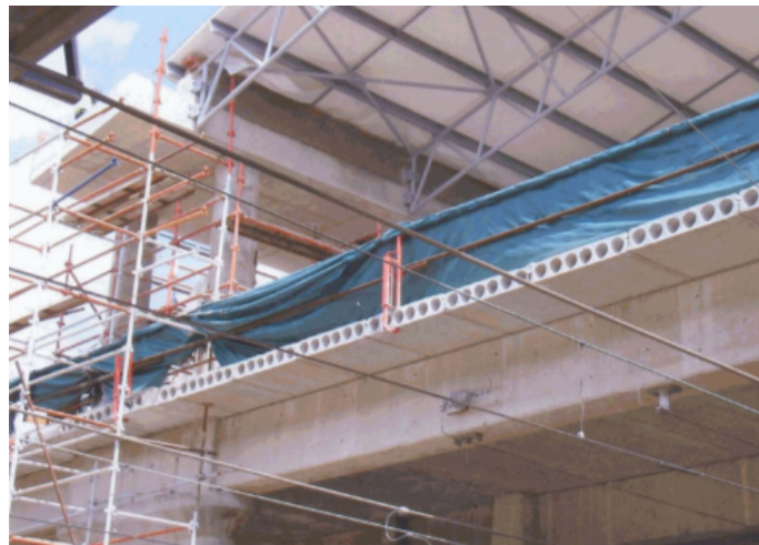
Figure 4.2: Pre-fabricated hollow-core slabs installed at the Orlando Station upgrade project (Civil Engineering 2010)
