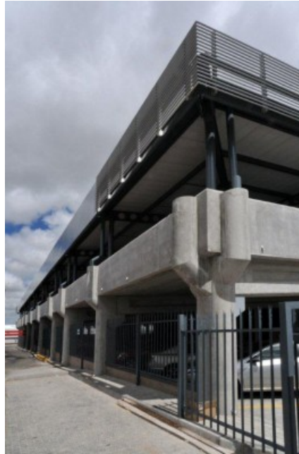
Figure 4.5: Precast columns, beams and floors used at the Honda Showroom (Concrete Trends 2011)
