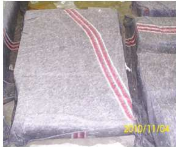
Figure B.2: Curing of flexural beams
