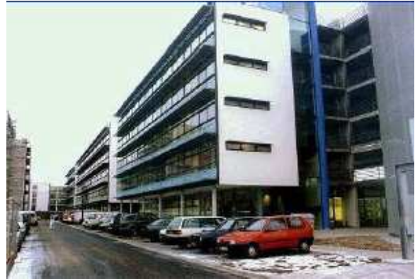
Figure 2.3: Vilbeler Weg office building, Darmstadt, Germany, 1997/1998 where almost 480 m 3 of RCA was used.
