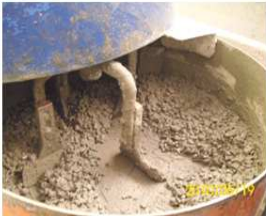
Figure B.9: Mixing of concrete
