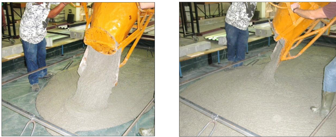
Figure 8.8 SCSFRC direct discharge from concrete bucket to flexural test slab mould
