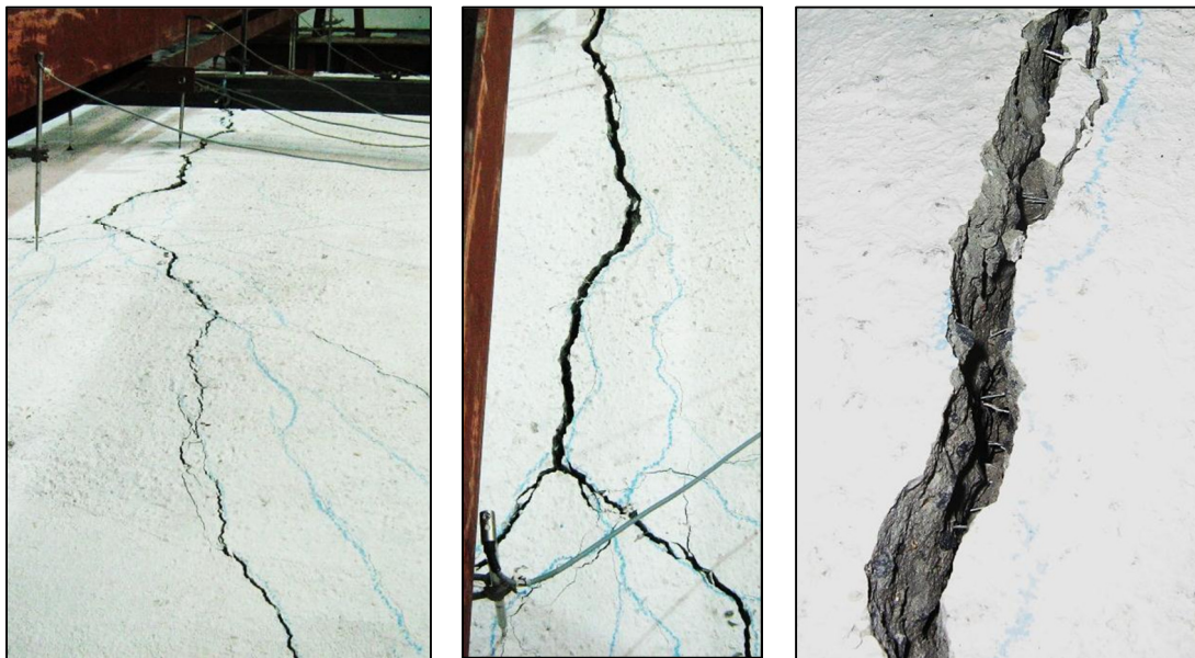
Figure 9.22 Hinge formation resulting from localised deflection softening
