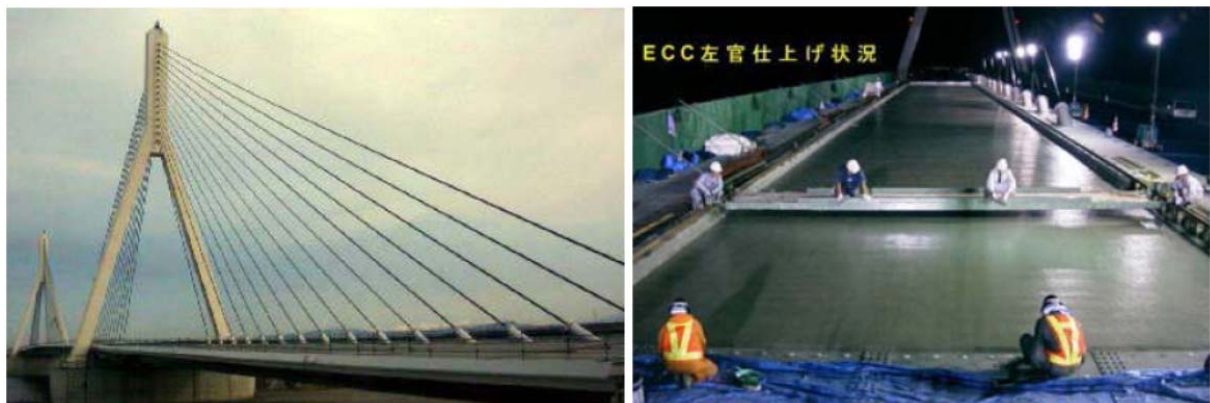
Figure 10 - Mihara Ohashi SHCC-Steel Composite Bridge (Courtesy of K Rokugo, van Zijl & Boshoff, 2008)
