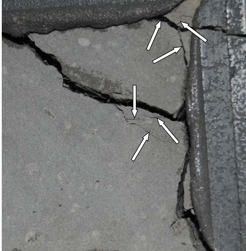
Figure 93 - Multiple crack formation on a specimen that has failed in biaxial tension (Point 12, Figure 3)
