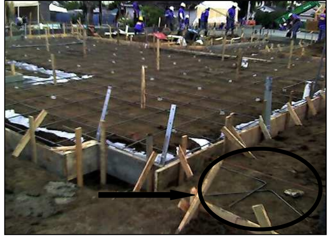
Figure 20: Rebar off-cuts on in-situ construction site (Crawford, 2003)
