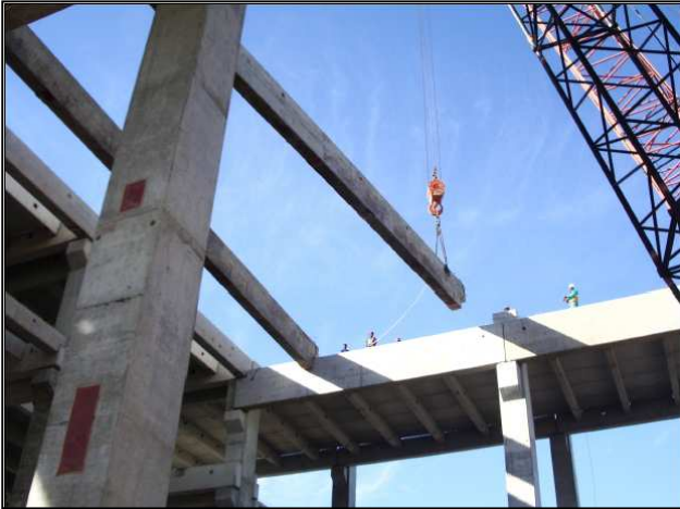
Figure 19: Placement of precast beam at VWSA paint shop in Uitenhage (Jurgens, 2008)
