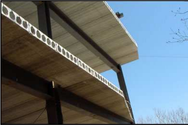
Figure 6: Hollowcore floor (Hollowcore, 2010)
