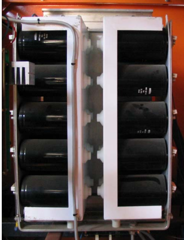
Figure 3.16 – Photograph of the Capacitor bank of one cell
