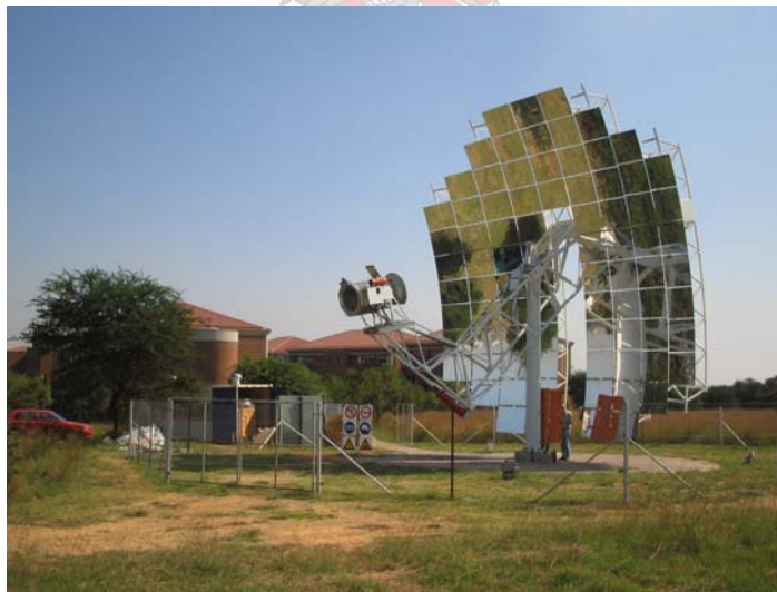
Figure 4-21: Picture of the SES with the DBSA in the Background
