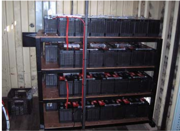
Figure 4-20: Picture of the Battery Rack Implemented at Site
