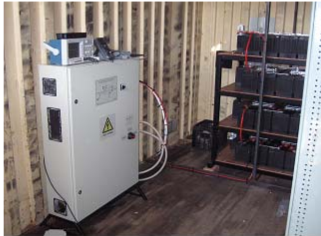
Figure 4-19: Picture of the Converter Implemented at Site
