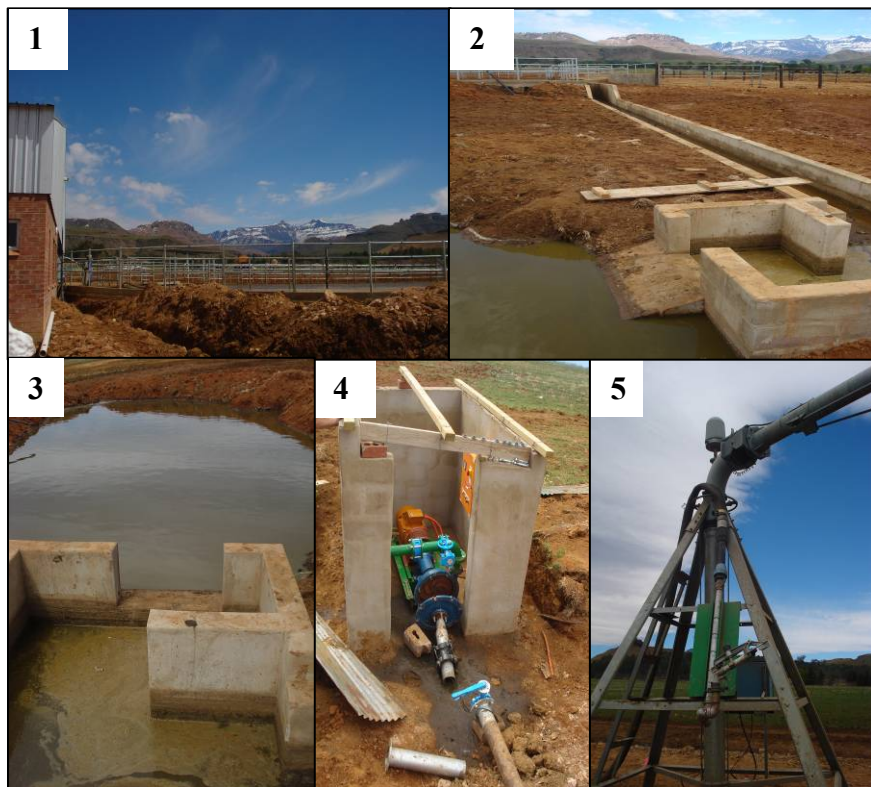
Figure 4.13: Bromley Farm system, showing separation of slurry using a lagoon system, followed by application onto pastures using an applicator gun mounted on a centre pivot.
