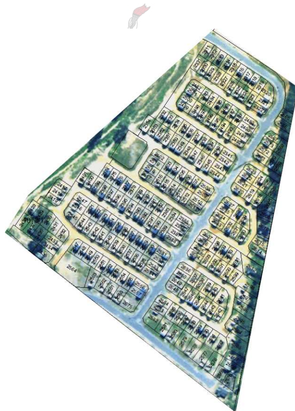
Figure K.1: Mooiwater Aerial View
