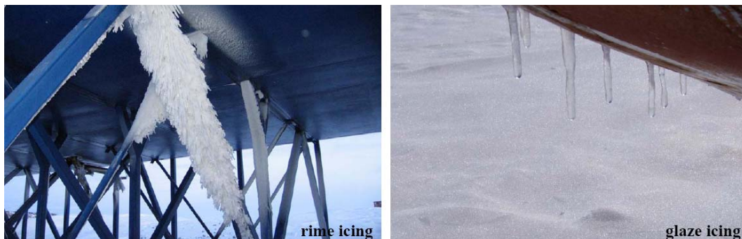
Figure B.2.1: Vesleskarvet icing (Stander, 2008)
