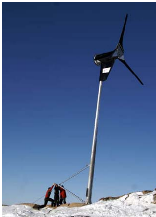
Figure 6.1: One of the Proven 6 kW rated wind turbines installed at the Belgium Antarctic Station, Princess Elizabeth (Anonymous, 2008c)
