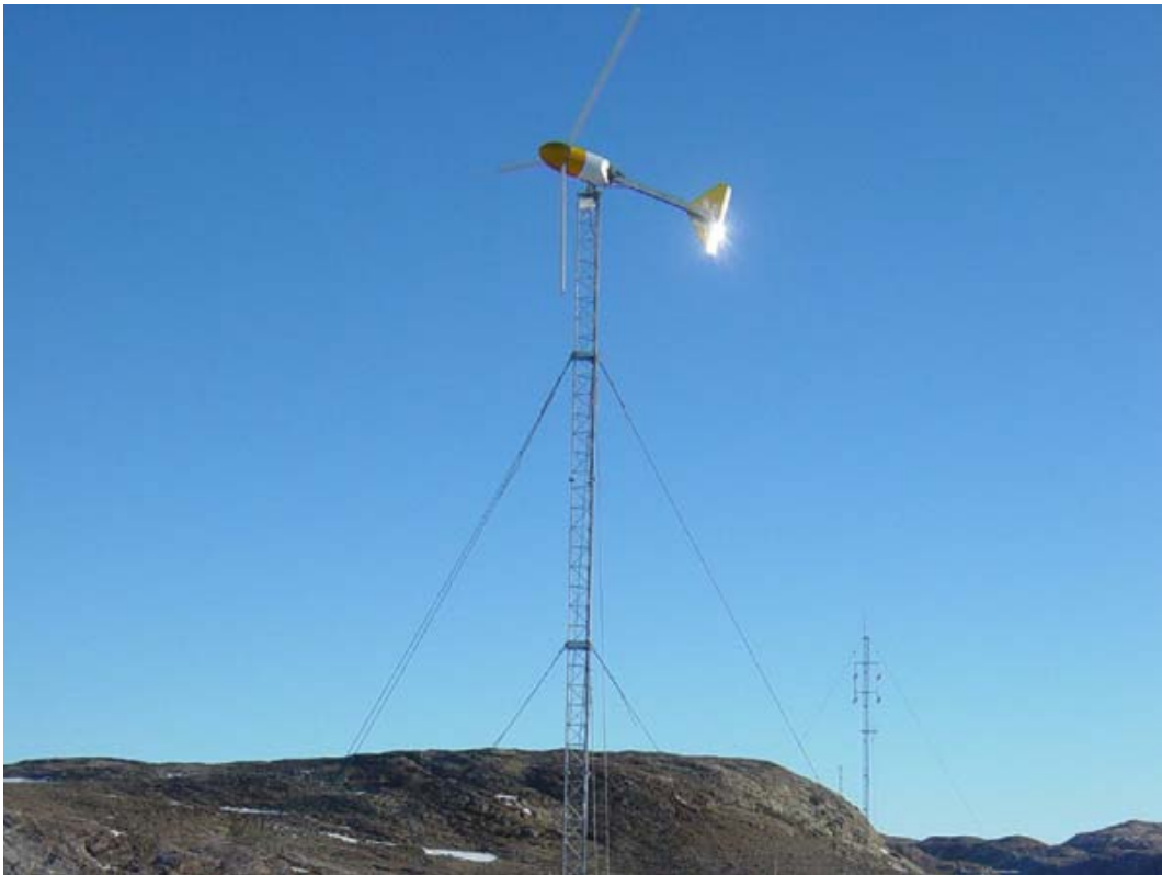
Figure 6.2: Bergey Excel-S wind turbine as installed at an Antarctic site (Bergey, 2008)
