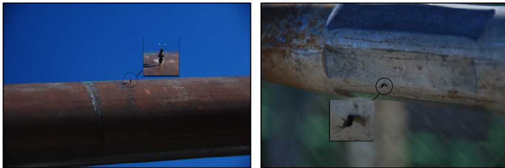
Figure E.5: Insects attracted to the positive DC conductors, fittings and and generator feed
