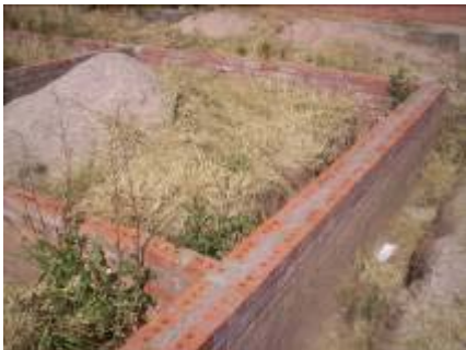
3) The foundation of a classroom that is incomplete due to lack of funds
