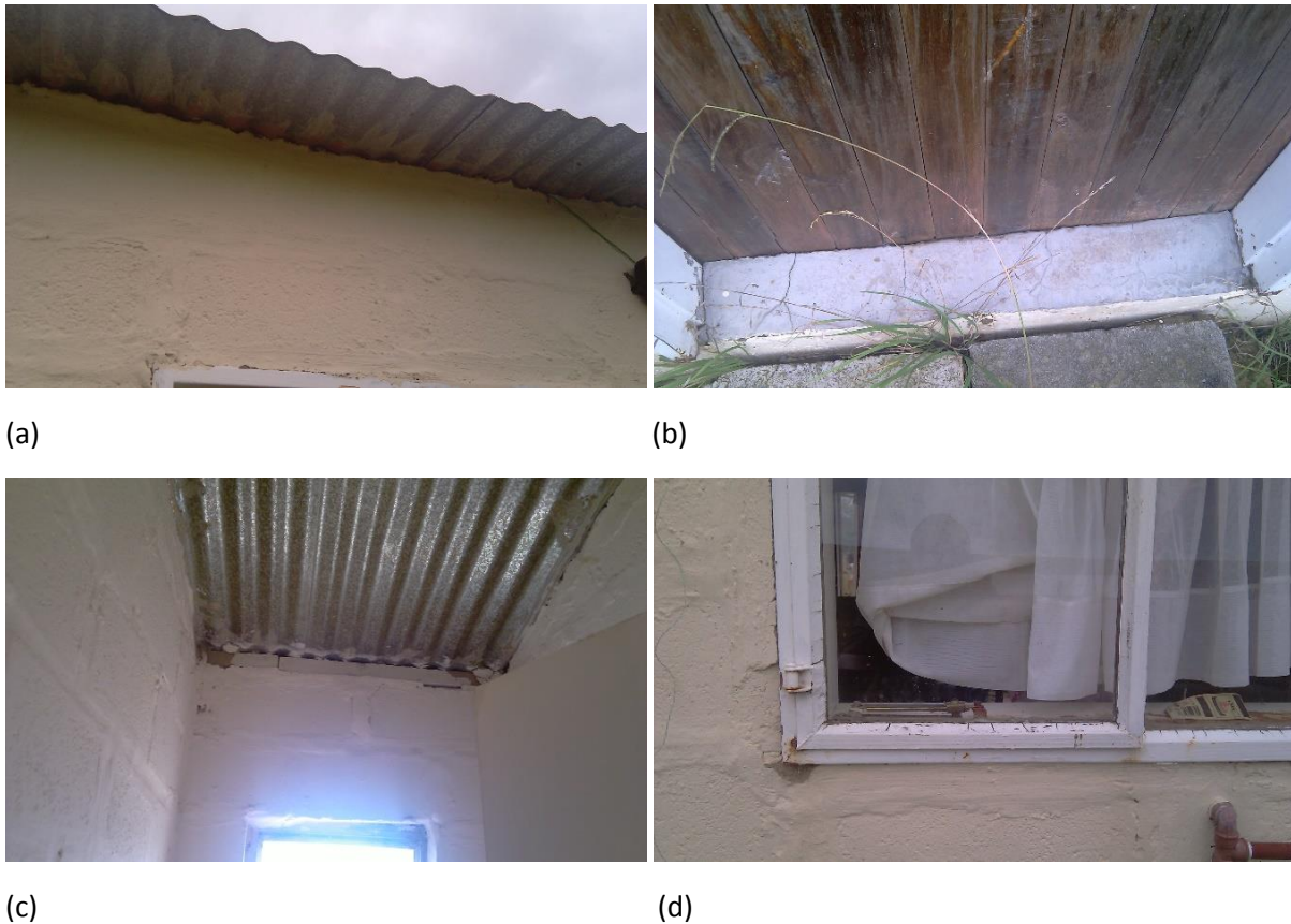
Figure 5.3: Sources of Air Leakage at the Studied House (Kelvin et al., 2017) (a) Cracks at the Outside Roof Perimeter (b) Cracks at the Sill of the Door (c) Cracks at the Inside Roof Perimeter (d) Loose Fitted Window Frame
