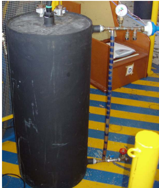
Figure 21 :- Tank with clear tube to monitor air volume
