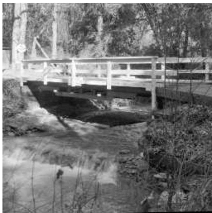
Figure A.3: Bridge
