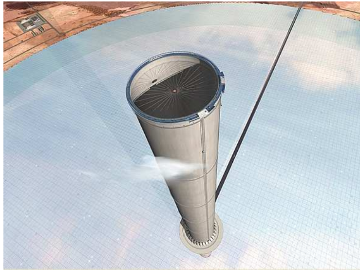
Figure 8-12. Spoked wheel concept visible at chimney tip [Schlaich Bergermann und Partner 2004].
