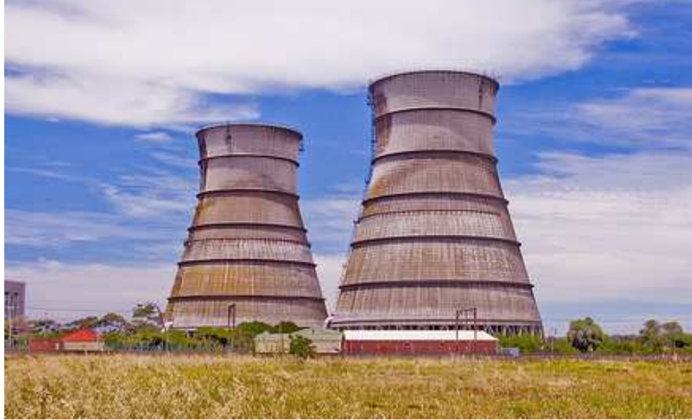
Figure 8-9. Circumferential stiffening rings in cooling towers [Internet 4 2008].
