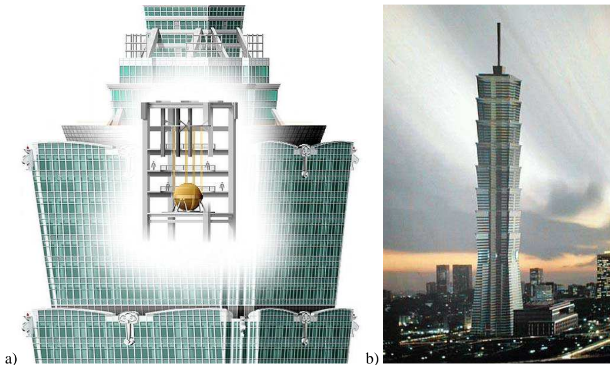
Figure 8-14. a) An example of a tuned mass damper [Internet 5 2008] as implemented in the b) super tall Taipei 101 building [Internet 6 2008].
