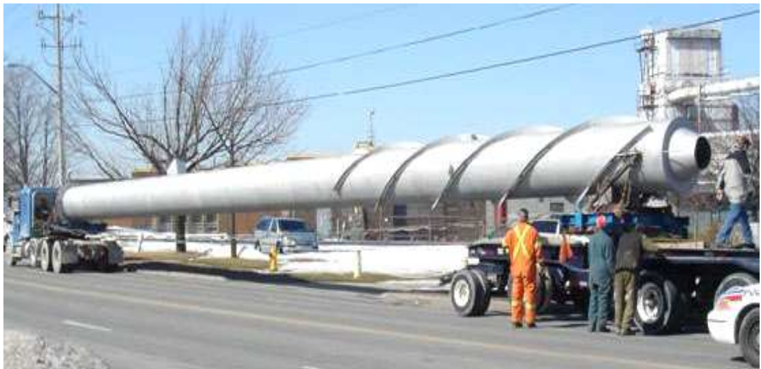
Figure 6-3. a) Systems for the manipulation of vortex induced vibration [Kumar et al. 2008] and b) an example of helical strakes wrapped around the upper third of a chimney stack in transit [Internet 1 2008].
