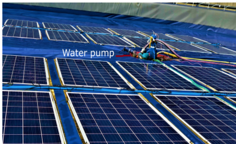
Figure 4.6: Solar modules on the floating canvas with a water pump located between the strings.
