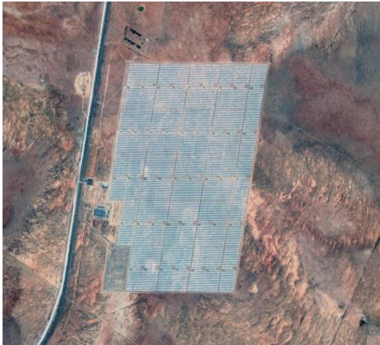
Figure 4.39: Aerial view of the Kalkbult solar PV power plant [141].
