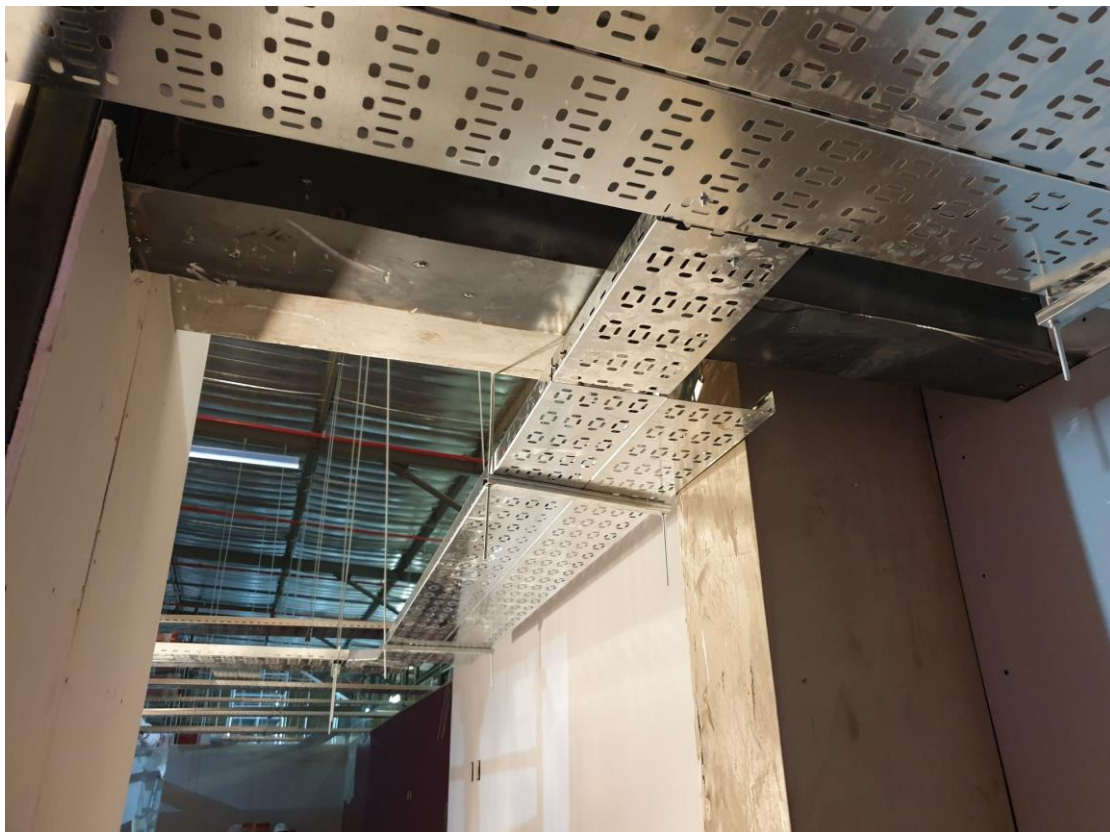
Figure 5-9: Electrical Services and Air Conditioning Services Second fix
