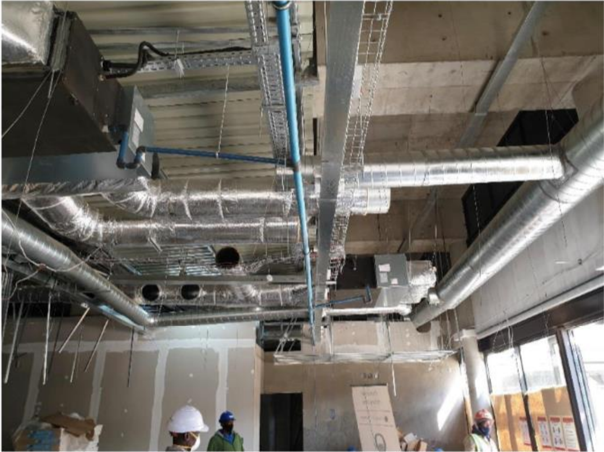
Figure 5-4: Heating Ventilation and Air Conditioning Duct Installation
