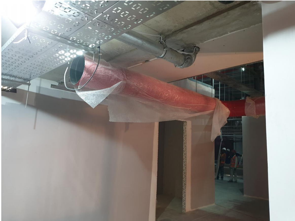
Figure 5-10: Electrical Services and Air Conditioning Services Third Fix
