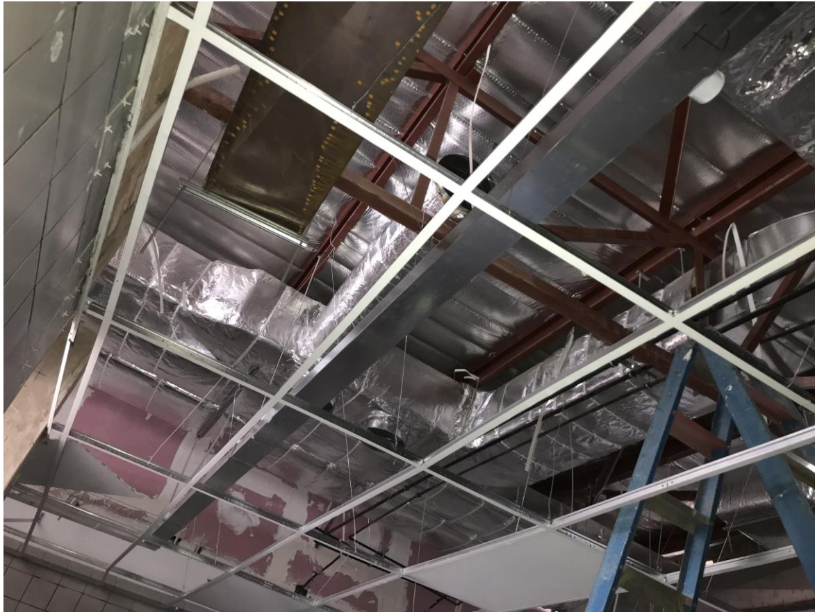
Figure 5-8: Electrical Services and Air Conditioning Services First Fix
