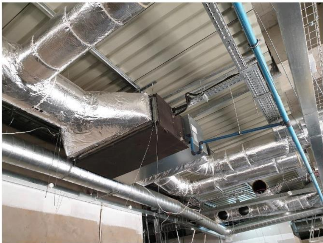
Figure 5-3: Heating Ventilation and Air Conditioning Duct Installation
