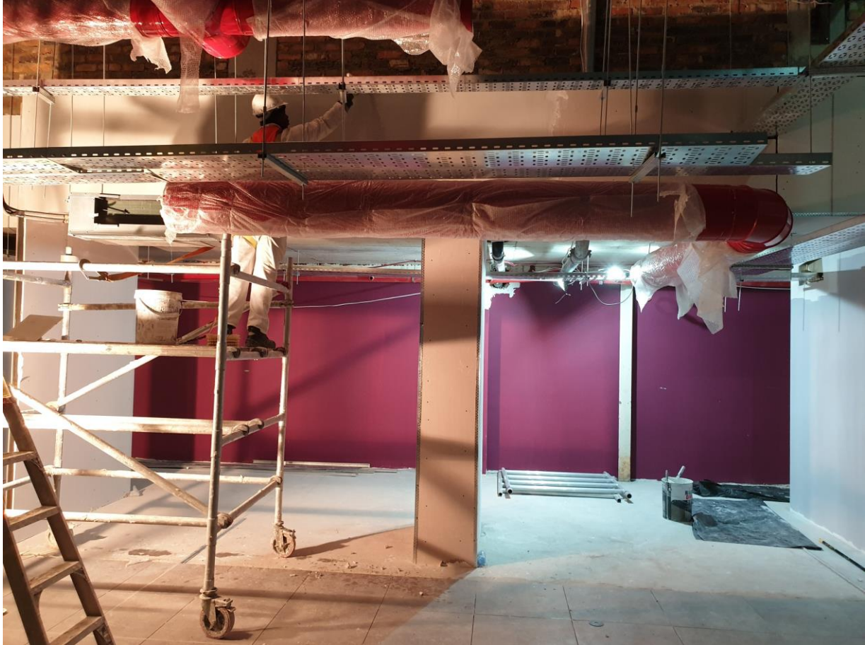
Figure 5-11: Electrical Services and Air Conditioning Services Third Fix
