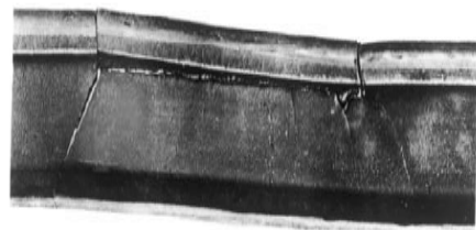
(f) Head/Web crack
