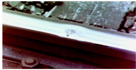
(b) Squat defects
