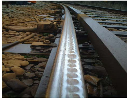
Figure 2.13: Rail corrugation (MORI et al. , 2010)
