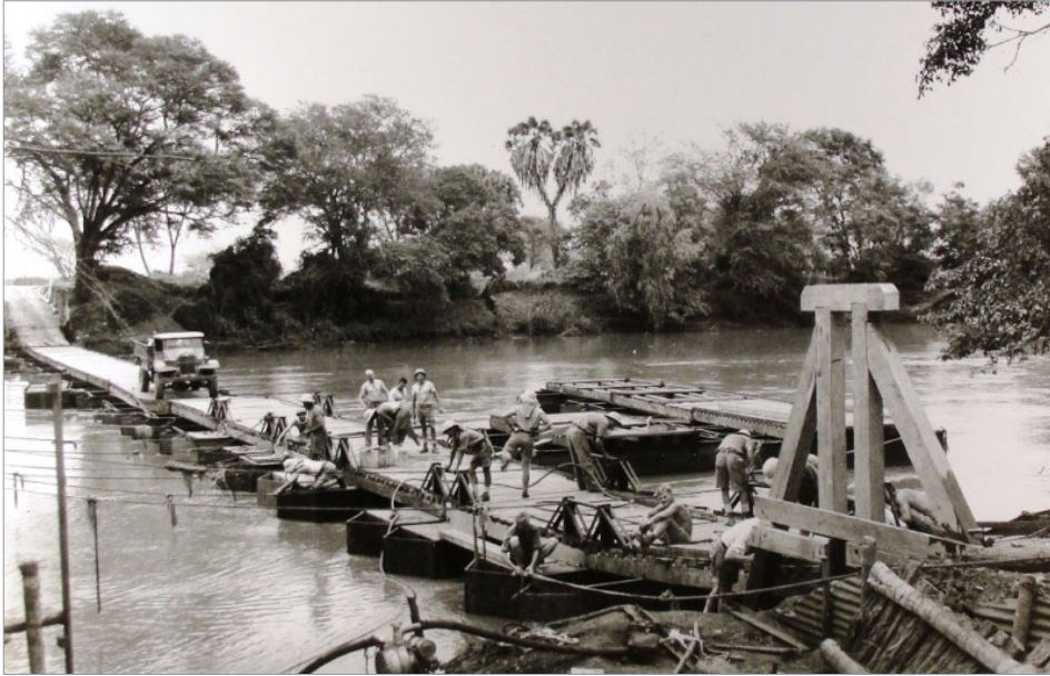
Figure 4.9 South African engineers successfully fording the Juba River 43
