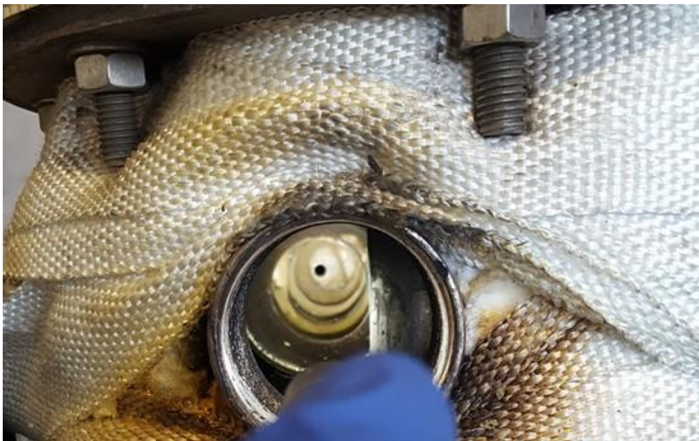
Figure 5.46: Melted plastic in exit pipe
