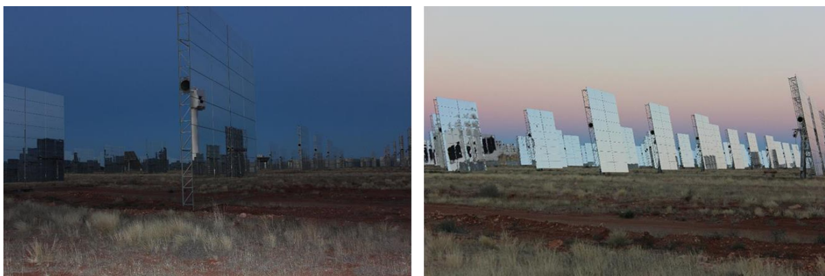
Figure 5.1 Khi Solar One heliostats positioned in a 90° vertical position at dawn (left).
