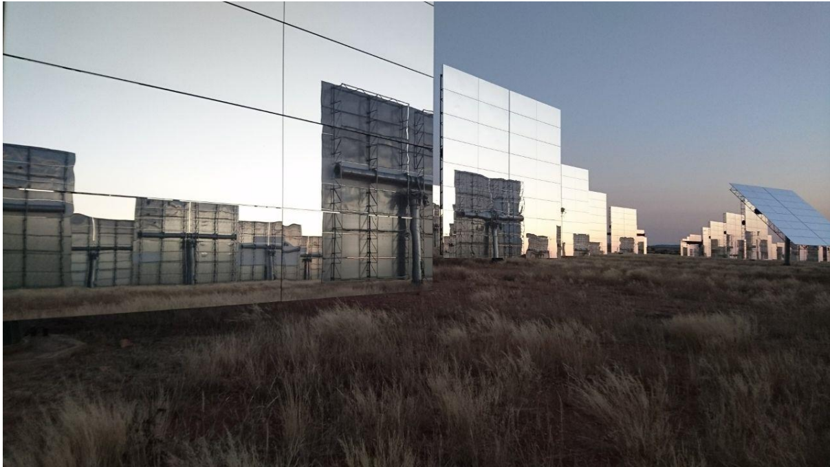
Figure 4.7 Khi Solar One heliostats positioned in a 90° vertical position during dusk.
