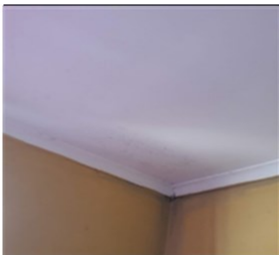
Figure 3: The ceiling in a RDP house
