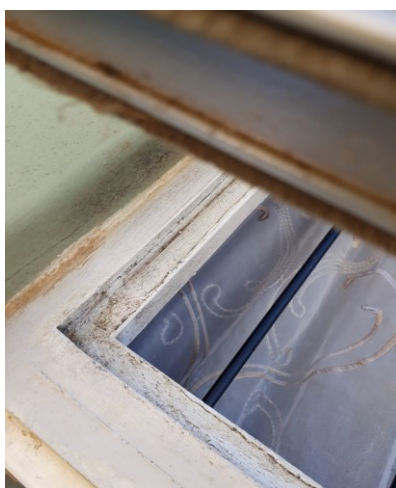
Figure 18: Mouldy window seals
