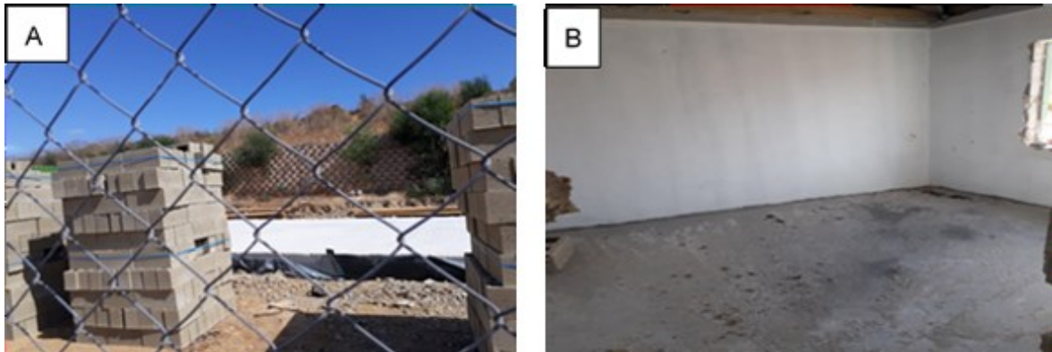
Figure 1: A) Concrete blocks used for building the walls and B) the concrete slab used for flooring
