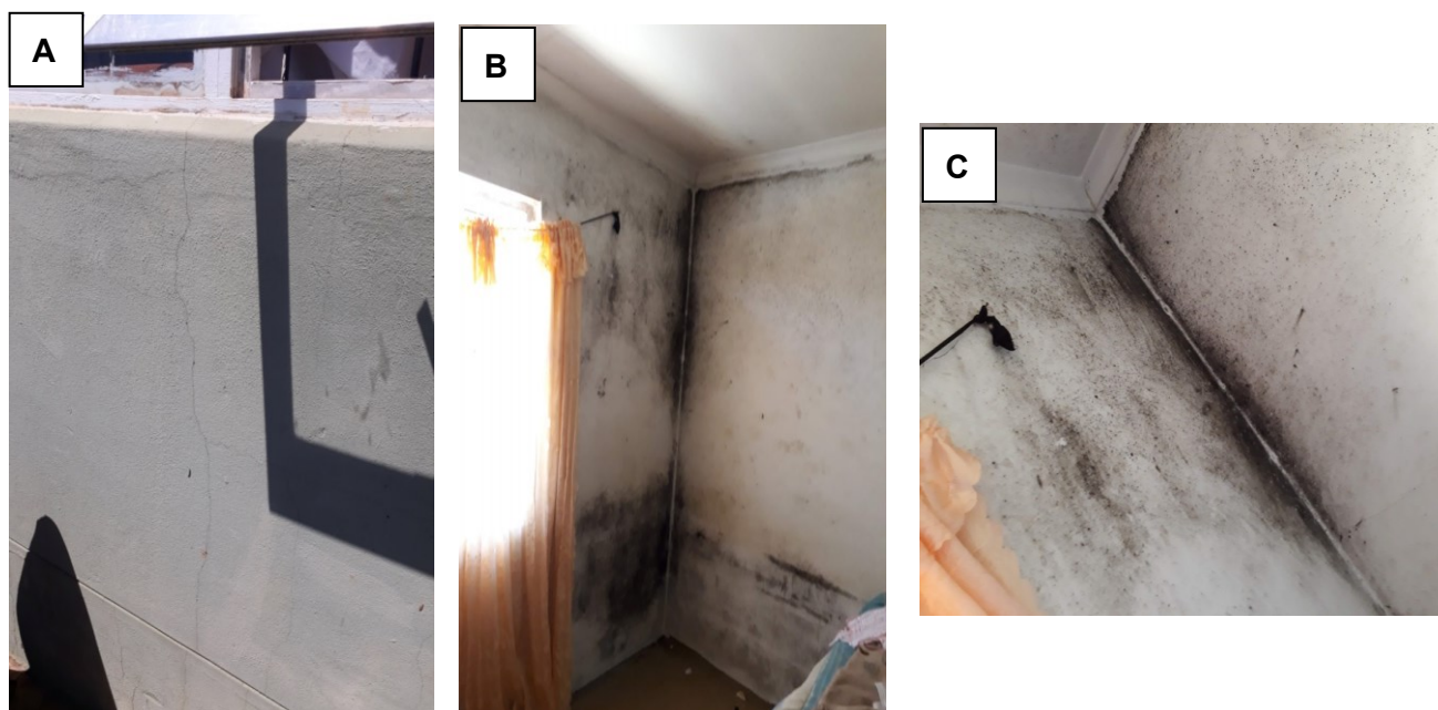
Figure 17: Examples of cracked (A) and mouldy (B, C) walls in RDP houses
