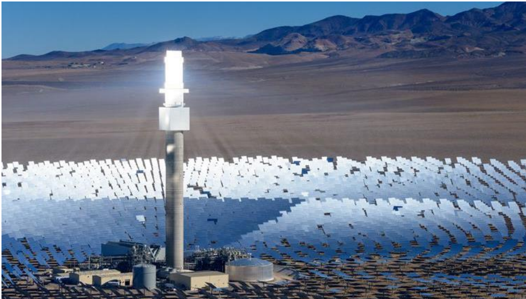
Figure 4-4: External receiver (Solar Reserve, 2017)
