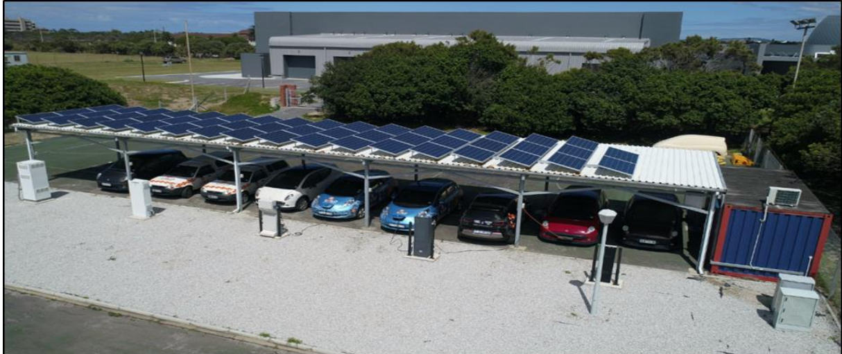
Figure 2.12: uYilo SmartGrid Facility
