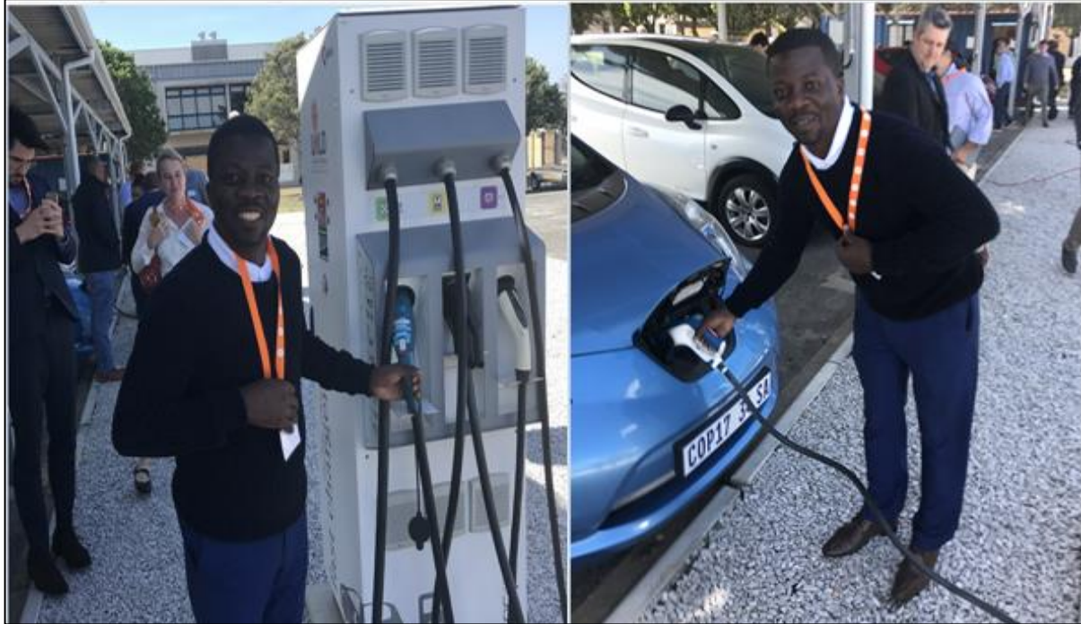
Figure 4.5: Workplace CHAdeMO Charging facility
