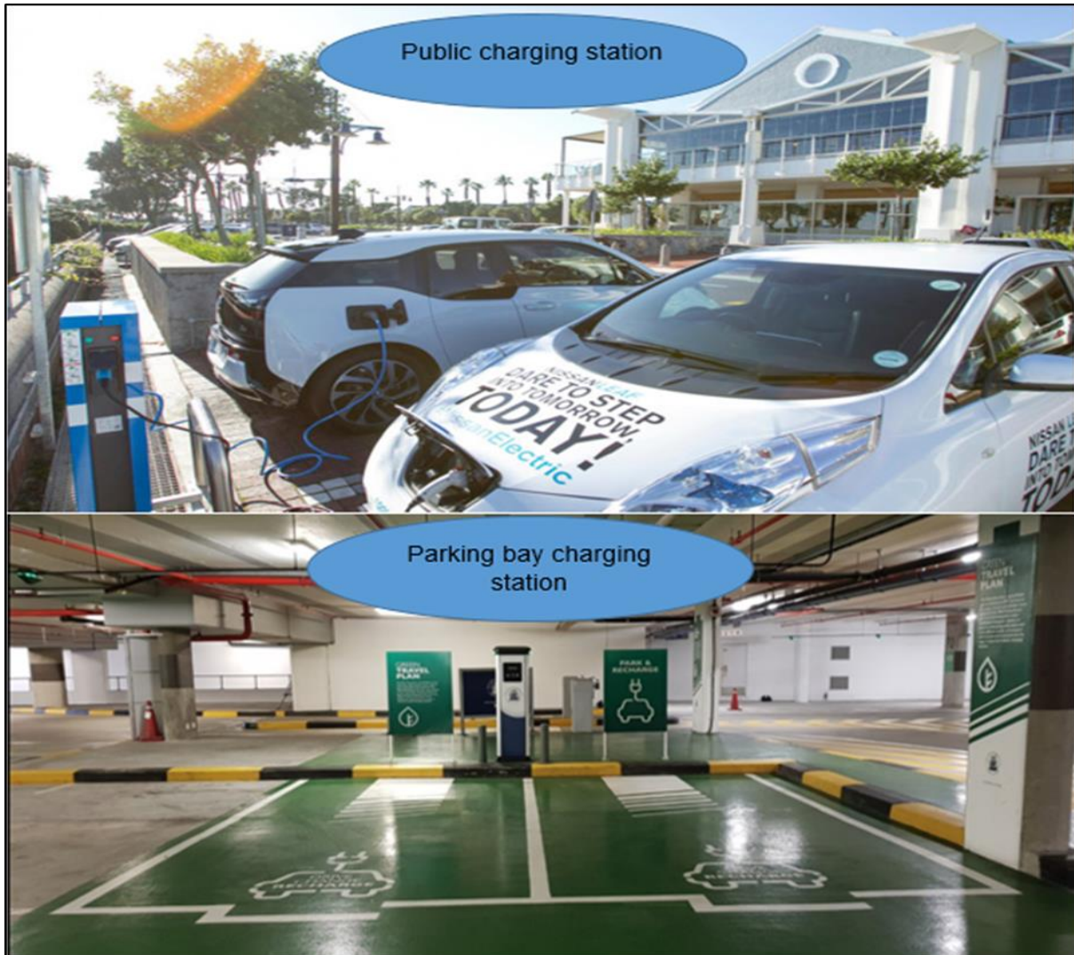
Figure 4.3: Public charging facilities in the Western Cape
