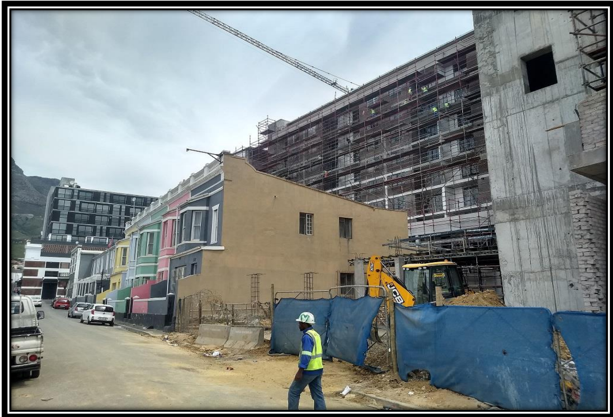
Figure 6. Gympie Street Redevelopment.
