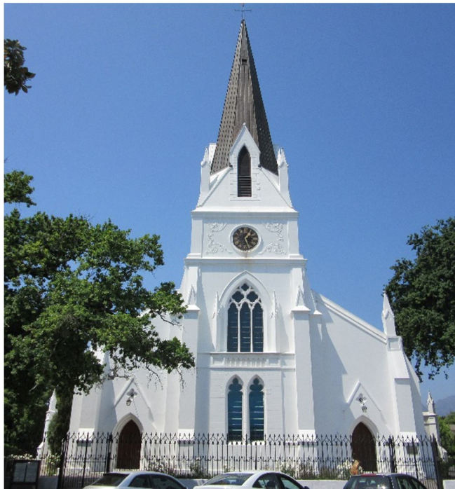
Figure 1: Current Moederkerk Building
