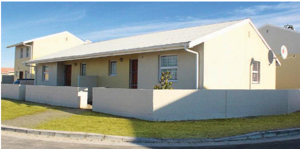
Figure 4.6: Single storey semi-detached two bedroom units – Harmony Village Source: CTCHC, 2013
