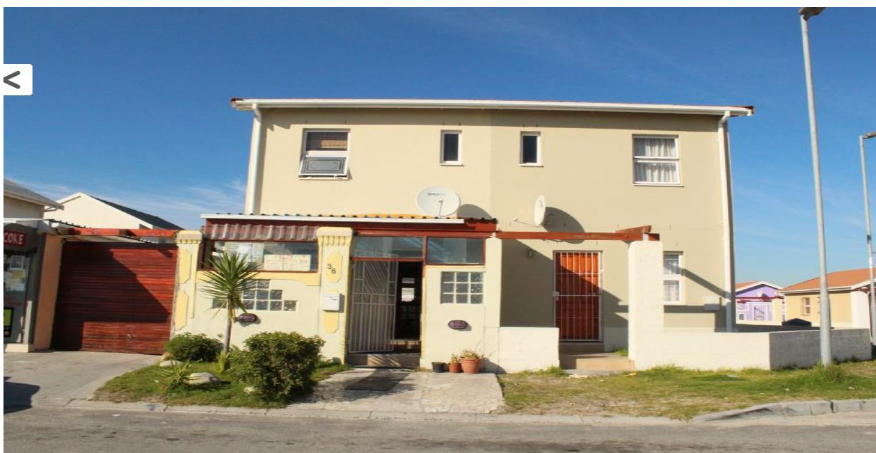
Figure 4.10: Double storey two bedroom units – West Cape Villas
