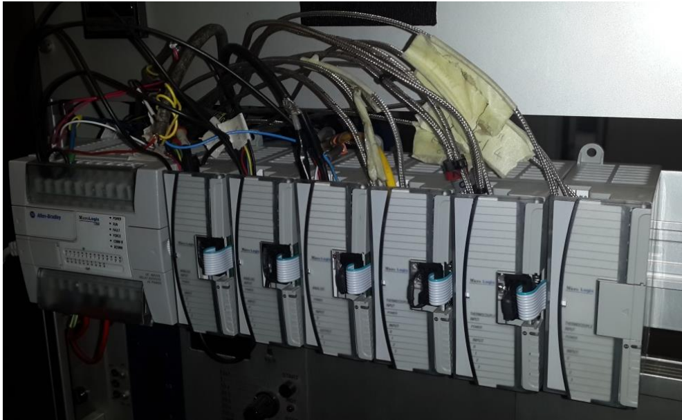
Figure 9: MicroLogix 1200 PLC and Expansion Modules
