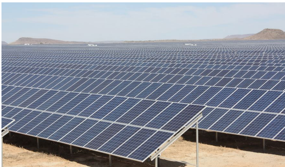
Figure 1.2: A stand-alone solar PV plant [4].
