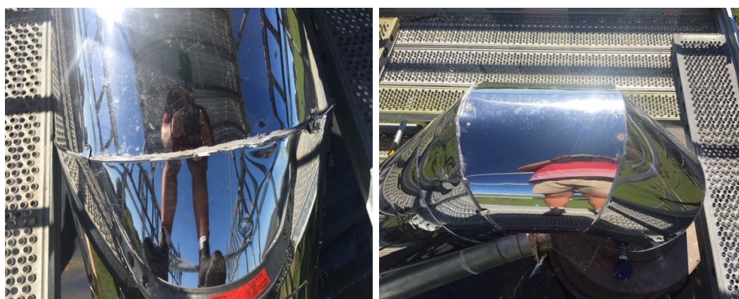
Figure 5.9: Leakage areas fixed
