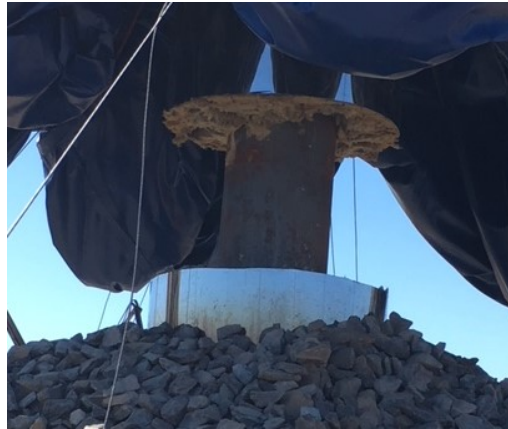
(a) Cladding and insulation removed
