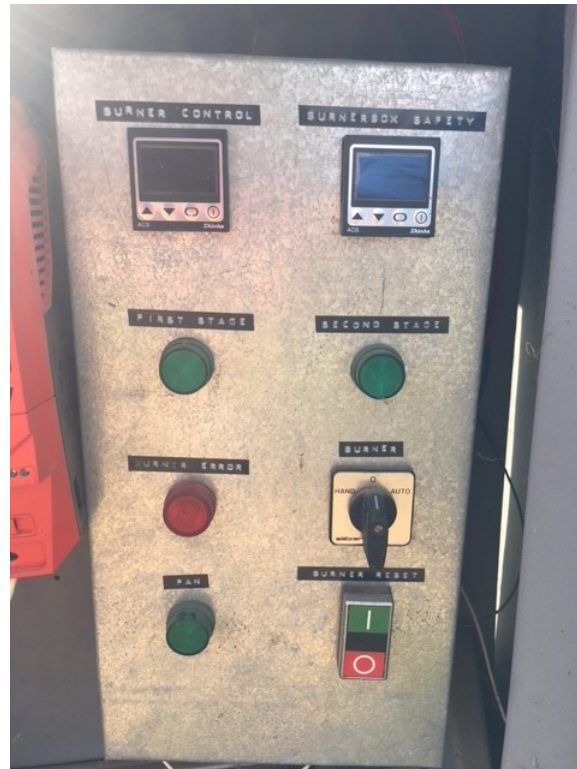
Figure C.12: Burner Control Panel
