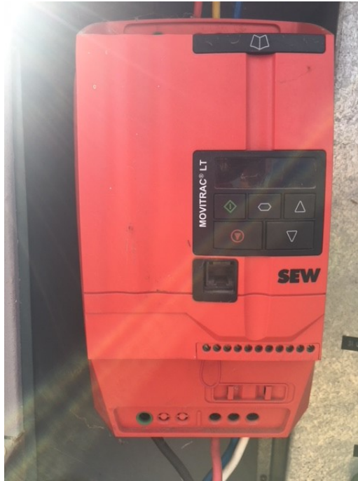
Figure C.5: VSD that controls the centrifugal fan
