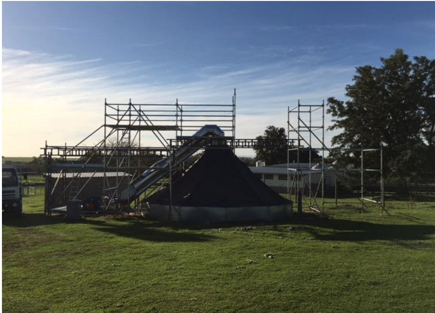
Figure 5.7: Scaffolding erected over the facility
