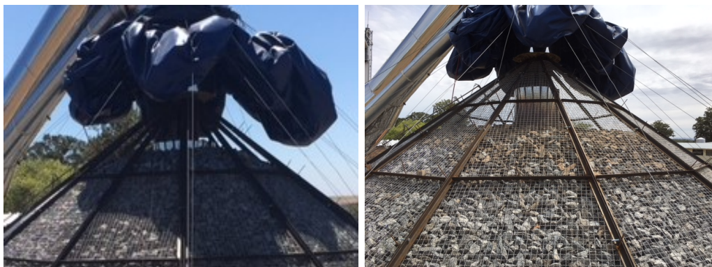
(a) Before shaping the rock bed
