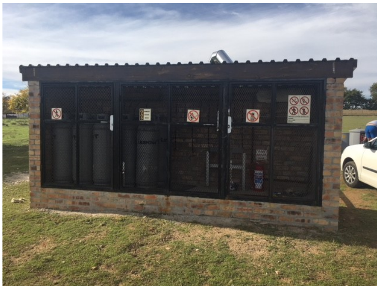
Figure C.7: Gashouse housing the LPG bottles
