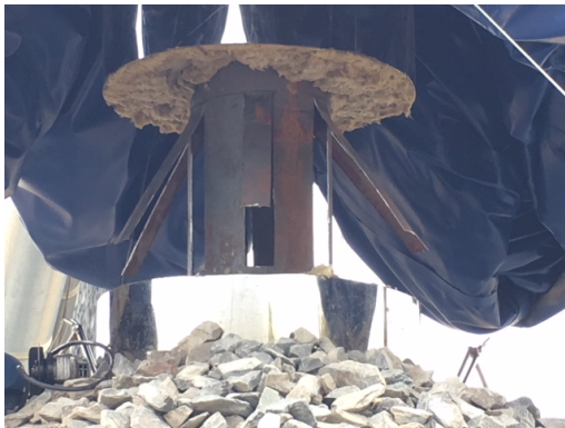
(b) Slits cut into steel pipe
