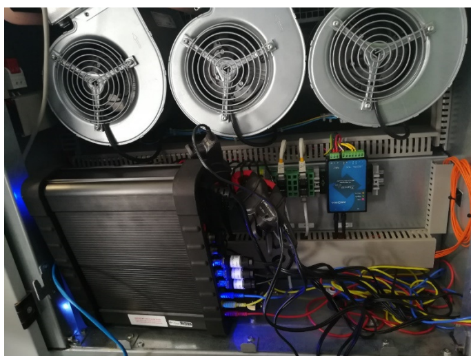
Figure 116: Physical current probes connections
