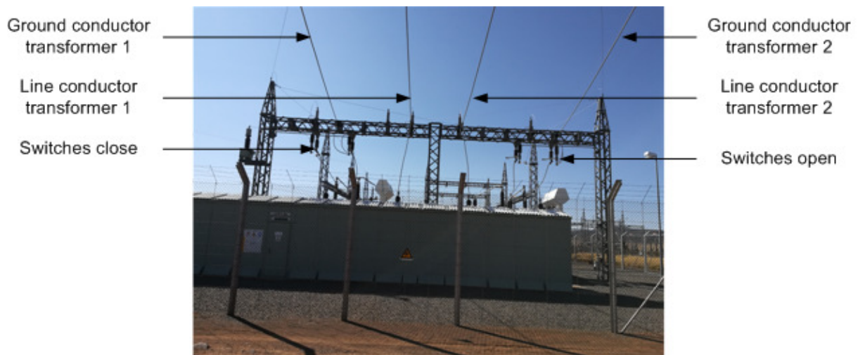
Figure 6: Traction substation with two transformers
