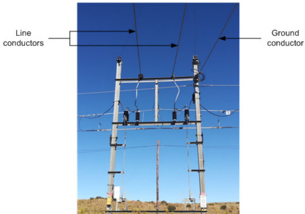
Figure 4: Connection between catenary and traction substation with one transformer
