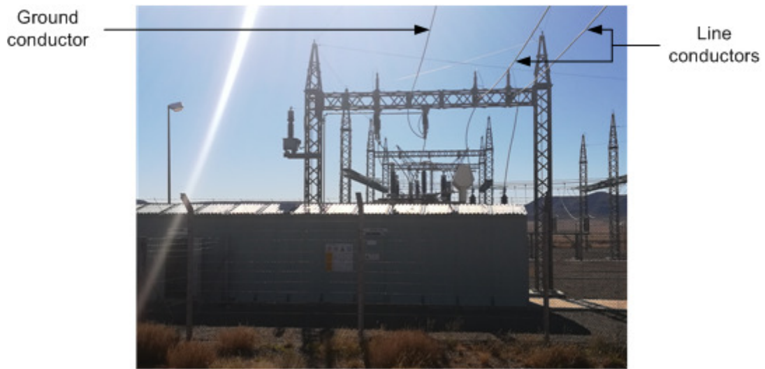
Figure 3: Traction substation with one transformer
