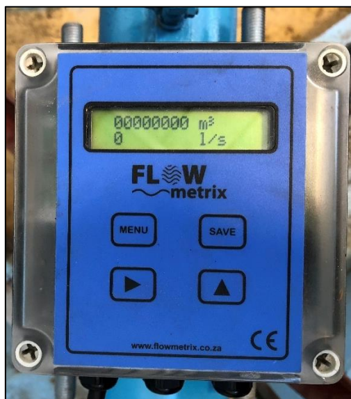
Figure 3.15: Reading Gauge of Flowmetrix Magflow DN100 Flow Meter
