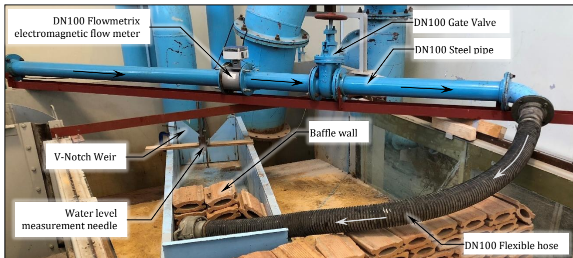
Figure 3.17: Flow Meter, Gate Valve and V-Notch Weir Setup
