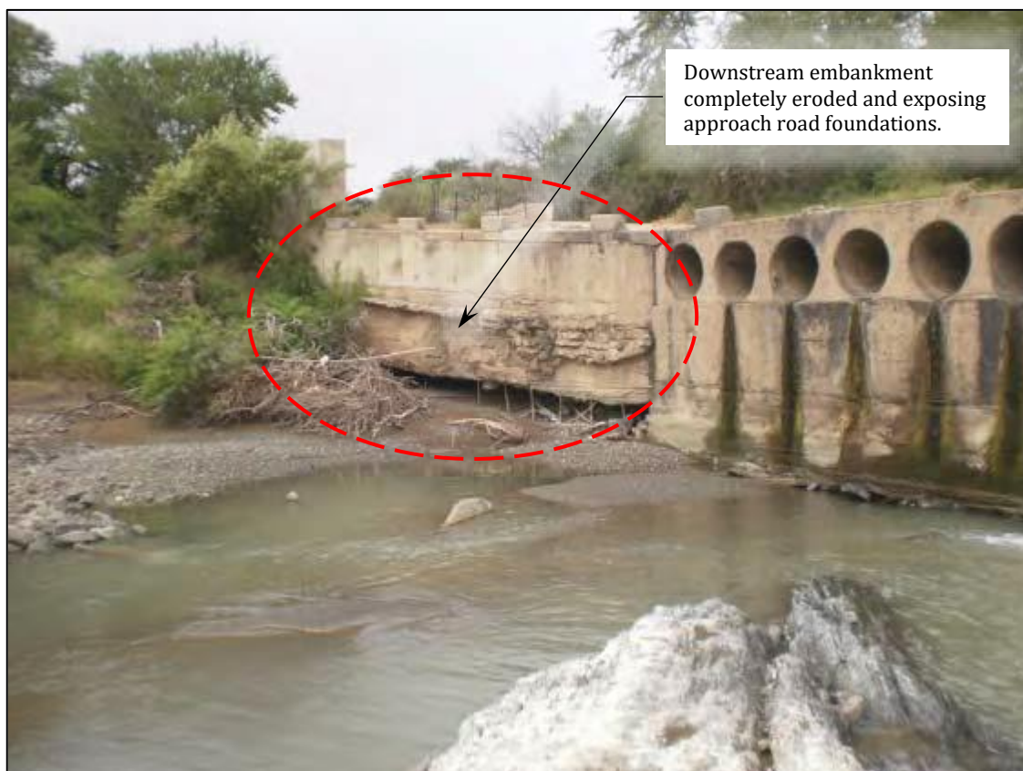
Figure 1.5: Embankment Scour Downstream of LLRC Approach Road (Photograph Courtesy of Hennie Maas, BVi Consulting Engineers)
