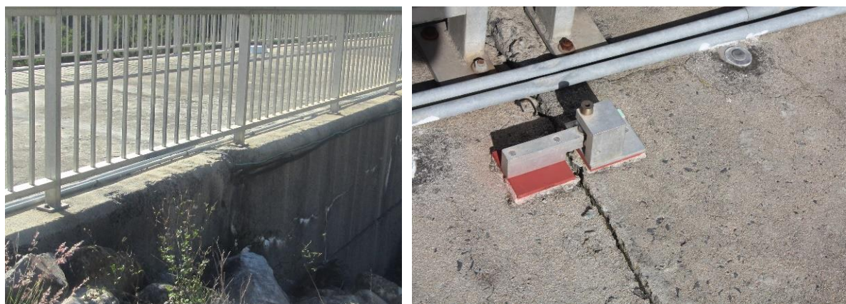
Figure 6-13. Displacement and cracking in the crest of the dam, a) sign of cracking in the upstream wall and b) vertical movements of the construction joint at crest at left flank.
