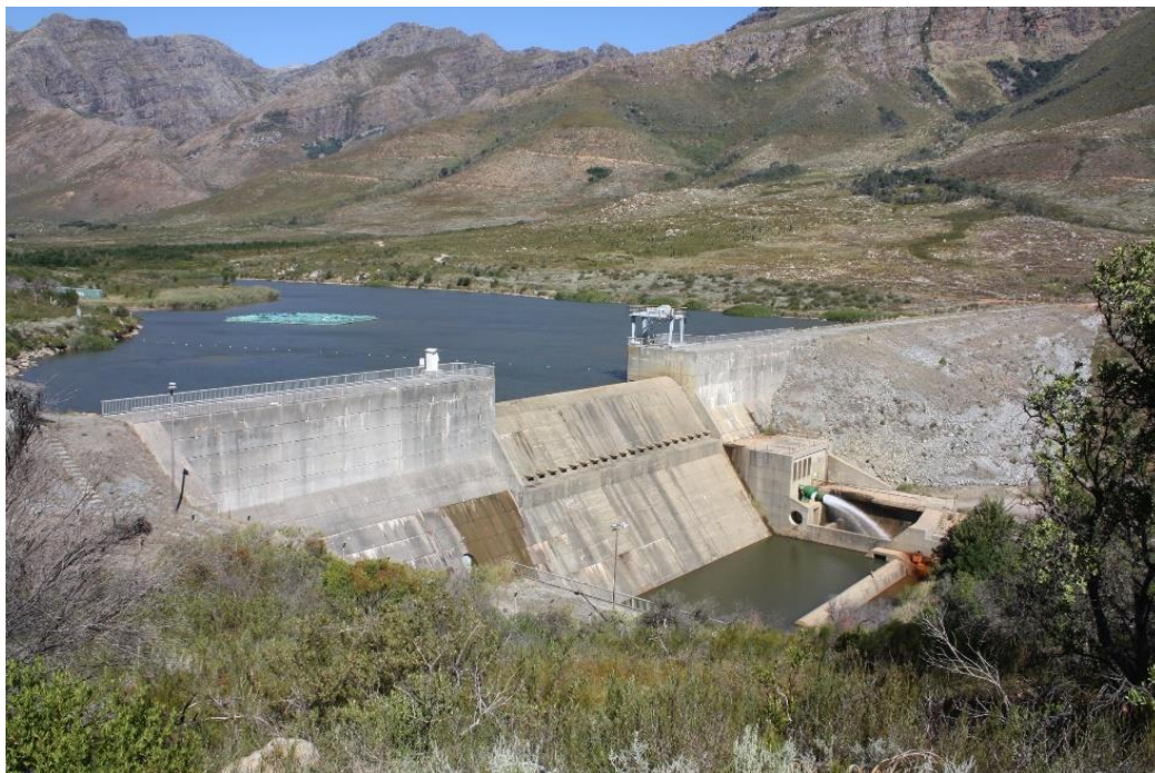
Figure 6-8. A perspective view of the Kleinplaas dam in the Jonkershoek River near Stellenbosch.
