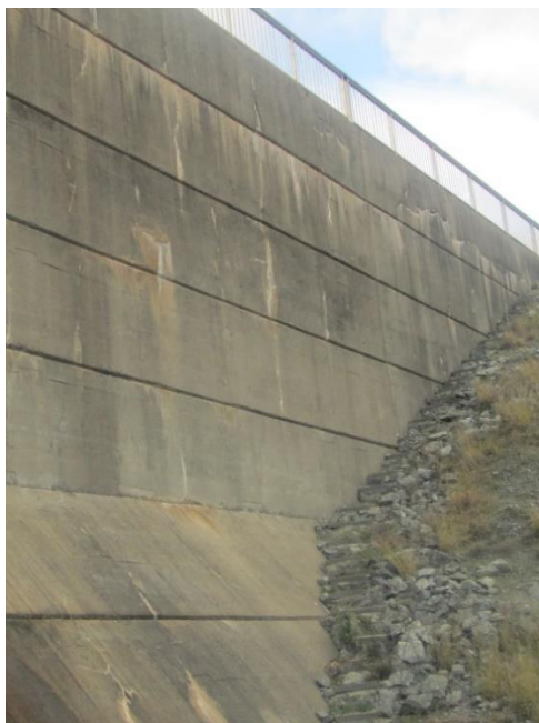
Figure 6-9. Perspective view from the downstream wall of the dam. Symptoms of leached reaction material through the micro cracks and joints are shown.
