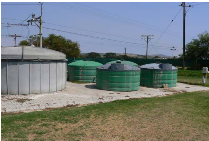
Figure 1.5: Biolytix Tanks - Lynedoch EcoVillage
