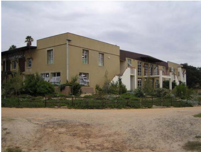
Figure 1.3: The Lynedoch Primary School and Sustainability Institute – Lynedoch EcoVillage
