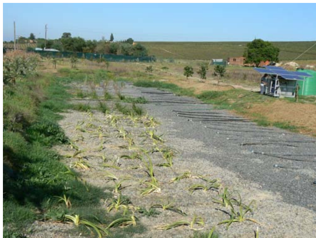
Figure 1.8: Surface area of the Vertically Constructed Wetland – Lynedoch EcoVillage
