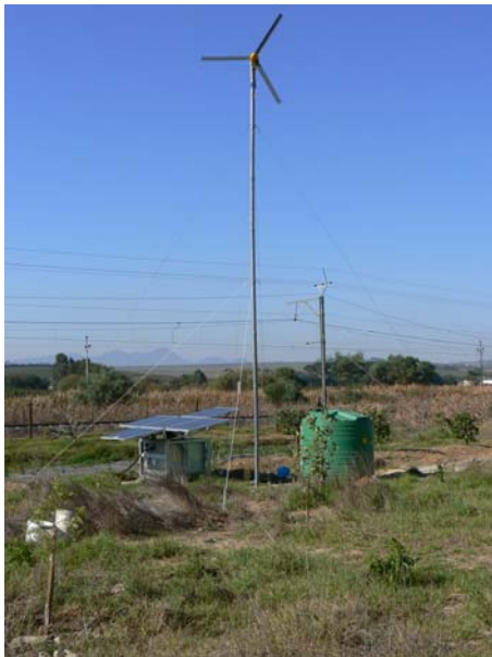
Figure 1.9: The Trunz Filter system, showing the windmill and solar panels - Lynedoch EcoVillage.
