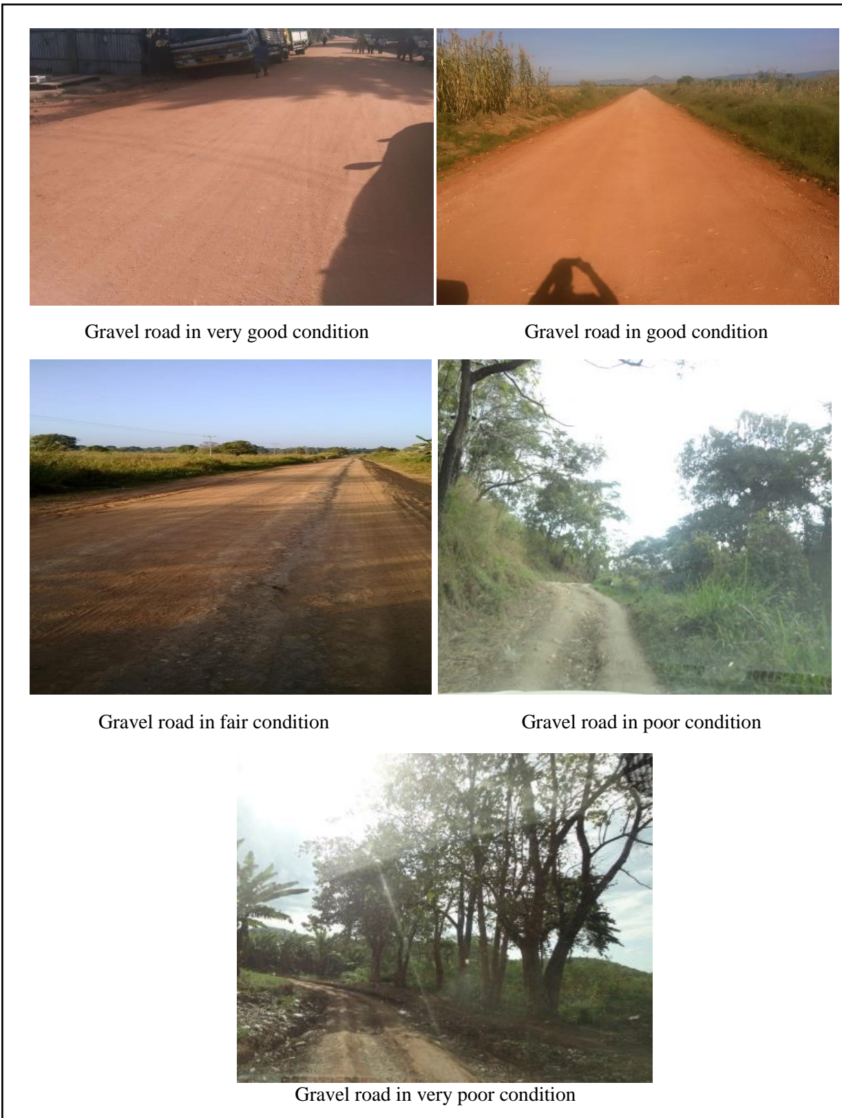
Figure A4.1: Pictures showing different condition of unpaved roads
