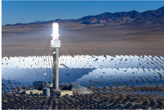
Figure 9: Central receiver system at Crescent Dunes (Solar Reserve, 2017).
