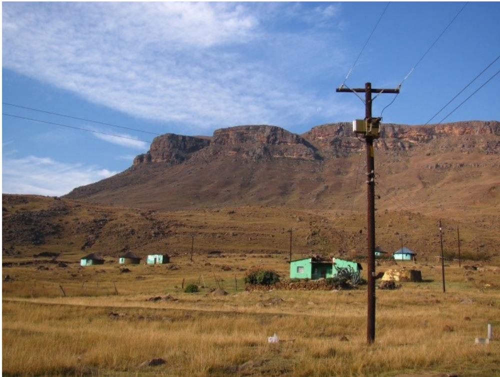
Figure 1: Example of a low population density, rural electrification installation with an overhead MV spur and single-phase LV feeder (near Tsolo, Eastern Cape, South Africa)
