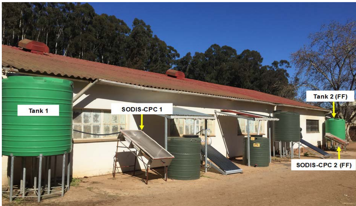
Figure 2.4: Rainwater harvesting systems located on Welgevallen experimental farm, Stellenbosch University, South Africa. The asbestos roof catchment area, is connected to the two tanks [Tank 1 and Tank 2 (FF)] via the conveyance system. Harvested rainwater flows passively from Tank 1 and Tank 2 (FF) into the SODIS-CPC-1 and SODIS-CPC-2 (FF) systems, respectively.
