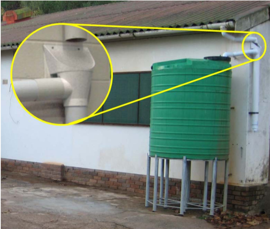
Figure A5: First flush diverter which is connected to the conveyance system between the catchment area and the rainwater harvesting tank (Tank 2).
