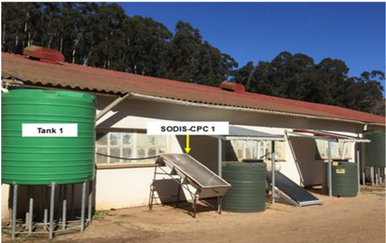
Figure 3.1: Rainwater harvesting systems located on Welgevallen experimental farm, Stellenbosch University, South Africa. The asbestos roof catchment area is connected to a rainwater harvesting tank (Tank 1) via the conveyance system. Harvested rainwater flows passively from Tank 1 into the SODIS-CPC-1 system.
