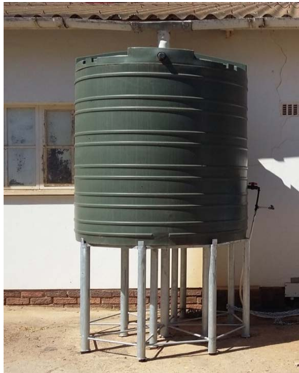
Figure 1.3: Above ground high grade polyethylene storage tank installed on a metal stand to enhance passive flow of the water from the tank.
