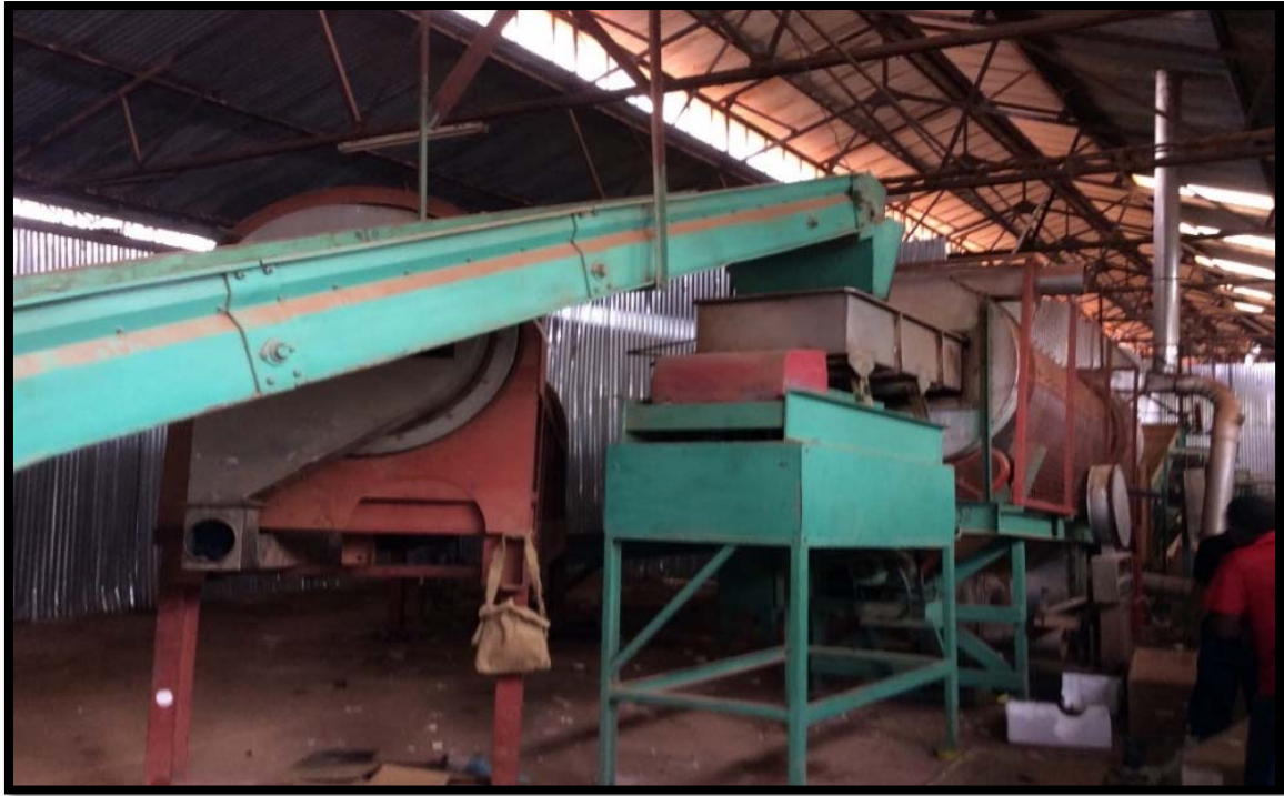
Figure 17: NGOMAT Tobacco Processing Plant Abandoned in Songea Municipality. 58
