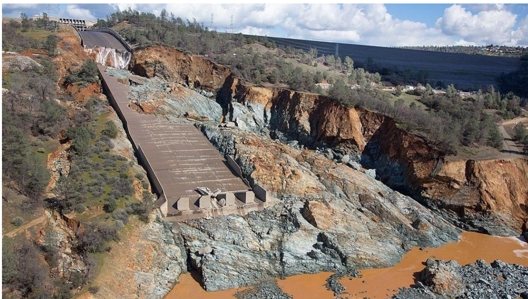
Figure 1.1: Oroville spillway damage, 27 February 2017, USA (Kolke, 2017).
