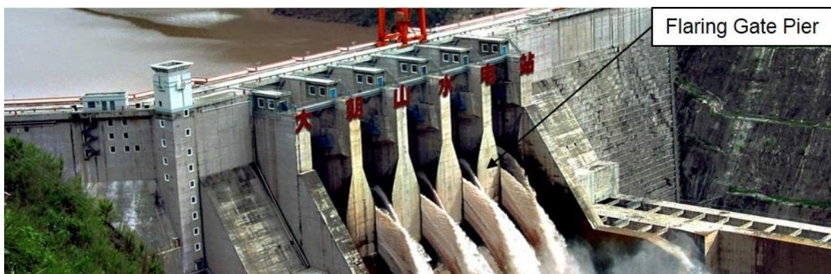
Figure 1.4: (i) Typical cross section through the Dachaoshan Dam (CHINCOLD, 2004) and (ii) photograph indicating the effect of the FGP on the spillway overflow (Hongta Group, 2017).
