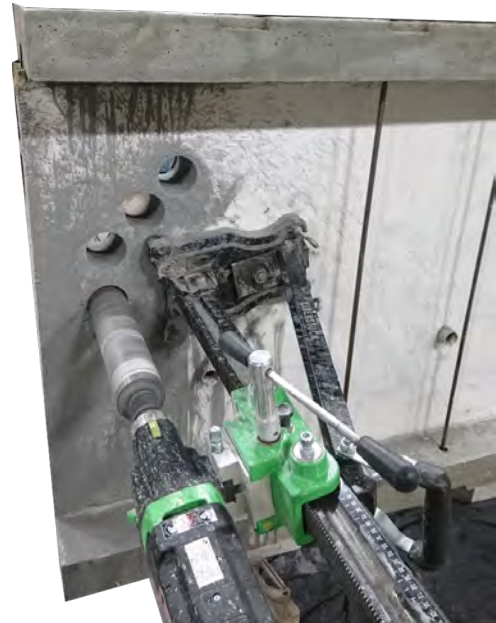
Figure 5.26: Core drill setup for LWFC walls
