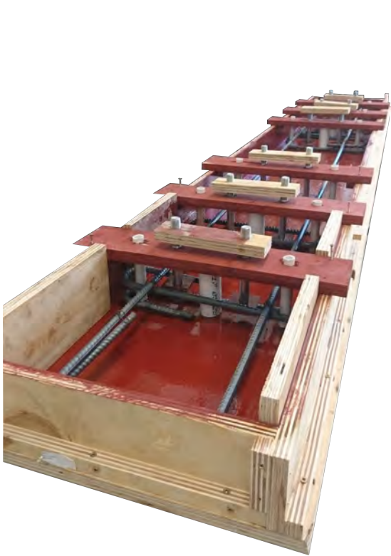
Figure 3.12: NWC mould and rebar before casting
