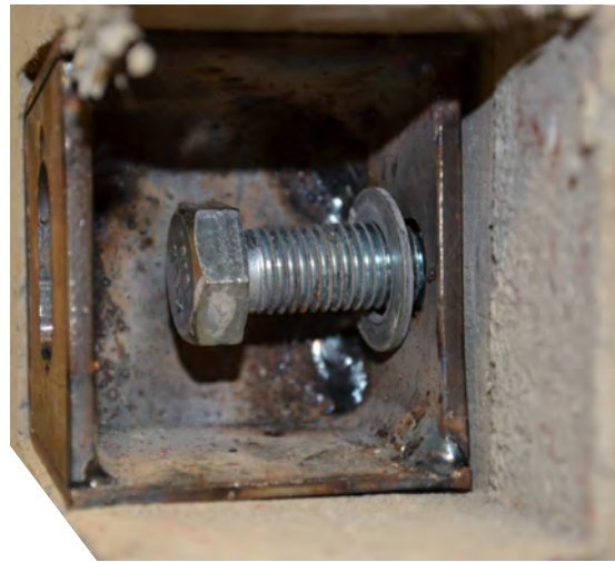
Figure 3.6: Vertical connection box showing slotted holes for adjustment and unfastened M16 bolt
