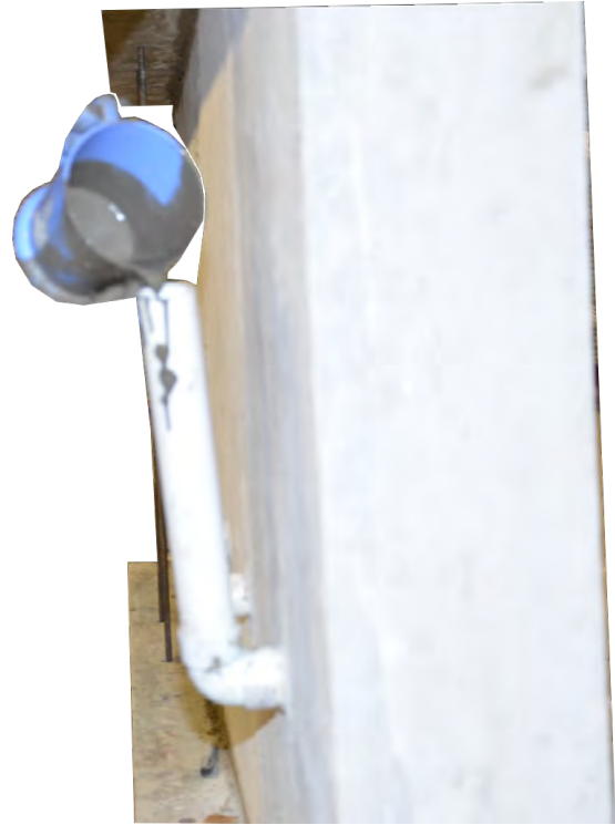
Figure 3.13: Grouting of lower grout connection between wall panels and "ground-slab"
