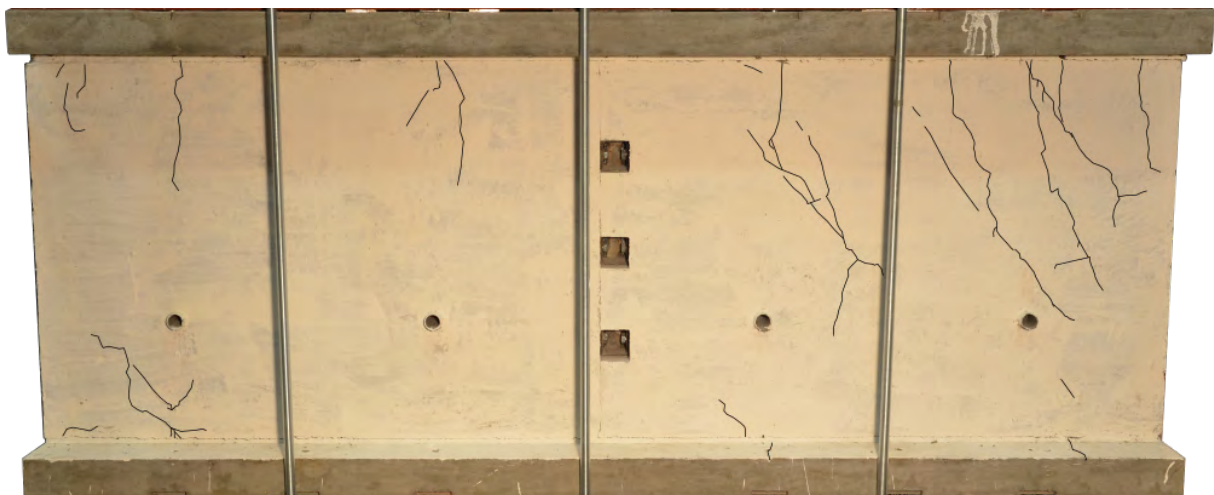
Figure 5.43: Final cracked state for physical test, PST 3
