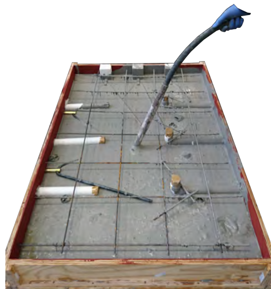
Figure 3.15: Flat casting and poker vibration of LWFC panel showing Y12 anchor rebar as well as mesh Ref. 193
