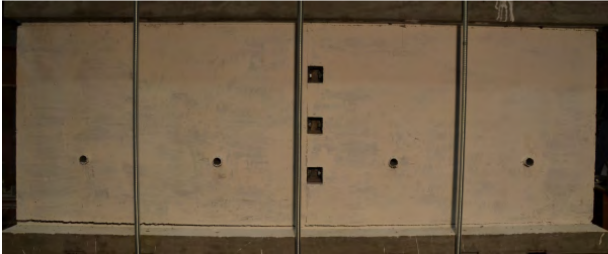
Figure 5.21: PST 3: Third nonlinear displacement region, visible slip at the upper horizontal connection.
