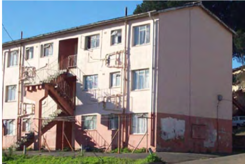
Figure 1.1: Typical unreinforced masonry low-rise residential building in the Cape Flats of South Africa (De Beer, 2016)
