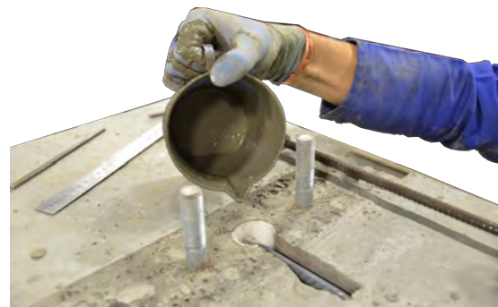
Figure 3.10: Grout process for "floor-slab" connection showing relevant details
