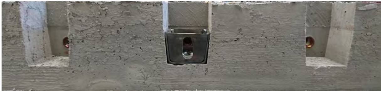
Figure 3.7: Connection box in moulded recess of LWFC panel, showing place for two additional connection boxes as well as embedded lifting anchors on this 1 : 3 scale wall
