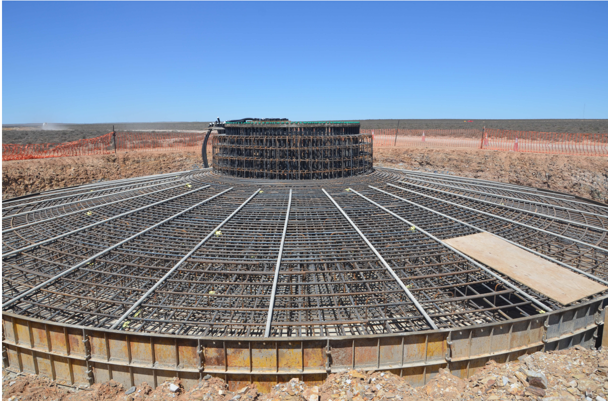
Figure 3.2: Fixed Reinforcement Steel
