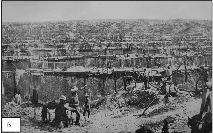
Figures 1 A & B - An illustration of the 5 meter roadways that was used to increase safety and effectiveness of individual mining operations at the Kimberley "Big Hole" Mine back in 1871 (Chilvers, 1938).
