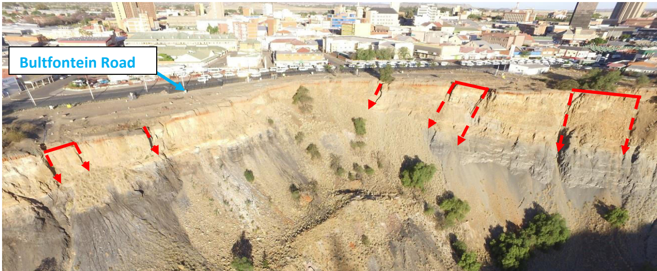
Figure 51 - Large-scale toppling blocks around the northern and northeastern side of the Kimberley Mine (closest to Bultfontein Road).
