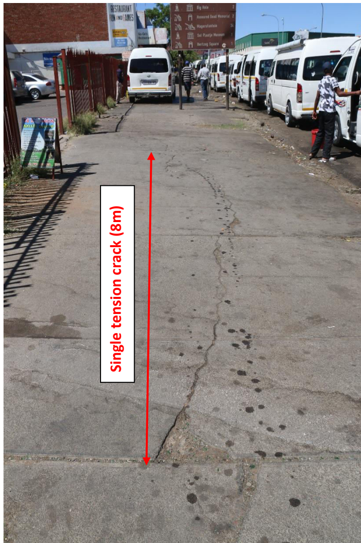
Figure 33 - A single tension crack on Bultfontein Road.
