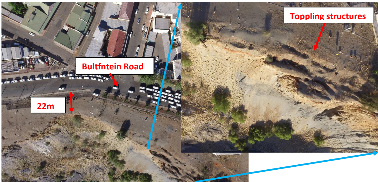
Figure 49 - Proximity of Bultfontein Road to the nearest edge of the Kimberley "Big Hole" Mine as well as large-scale toppling structures on the northeastern side of the pit.
