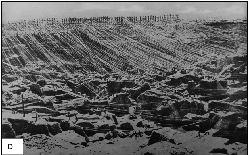
Figures 1 C & D - This was the preferred method of mining before implementation of wooden platforms / scaffoldings (also commonly referred to as "stagings") (Theodore, 1893)
