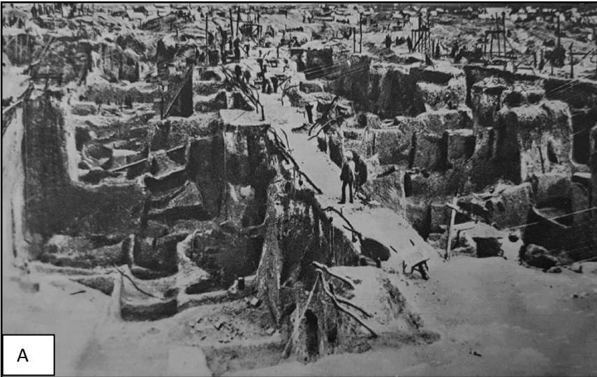
Figures 1 A & B - An illustration of the 5 meter roadways that was used to increase safety and effectiveness of individual mining operations at the Kimberley "Big Hole" Mine back in 1871 (Chilvers, 1938).
