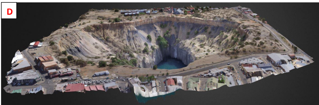
Figure 62 - 3D model of the west facing sidewall of the Kimberley "Big Hole" Mine.
