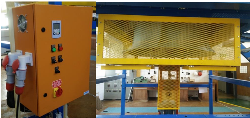
Figure 4-9: Varispeed 15 kW variable speed drive (left) and the safety screen (right)
