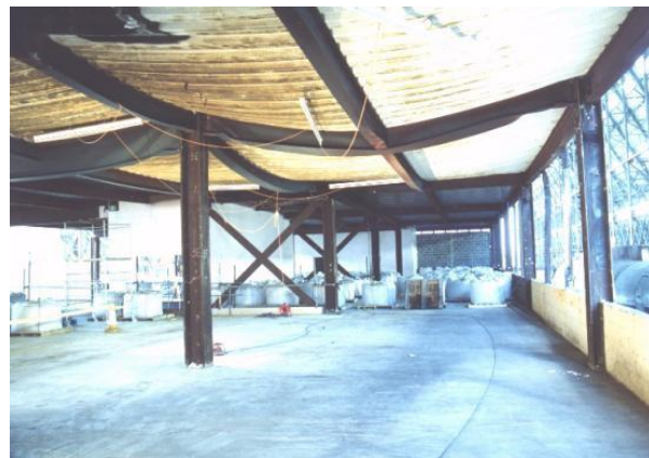
(b) Beams from the Cardington tests showing severe midspan deflections, and web buckling close to supports (Lamont, 2001)
