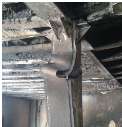
(a) 'Squashed' steel column (courtesy of Ali Moradi)
