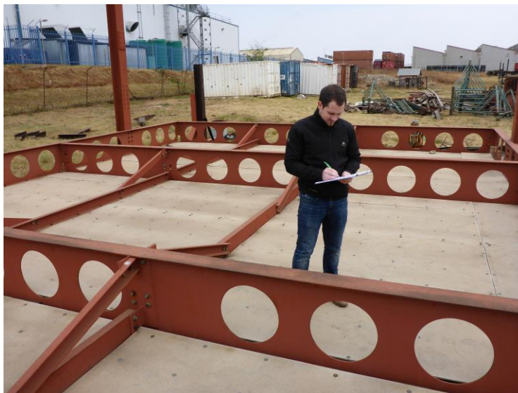
Figure 3.4: Hendrig Marx at the site of the prototype cellular beam structure (CBS)
