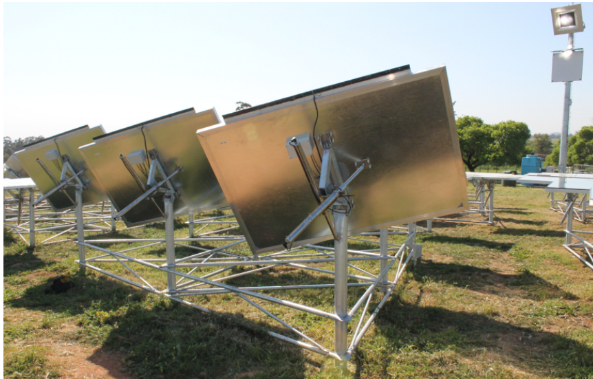
Figure 9.7: Sandwich type facets installed at the Helio100 field
