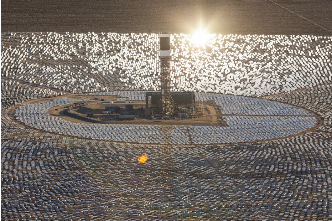
Figure 1.1: Ivanpah solar power plant in the Mojave Desert, California (Bright-Source Energy Inc, 2016). This plant uses around 173 500 software operated heliostats to follow the sun's trajectory with more than 300 000 mirrors, spanning over 14.2 km 2 .
